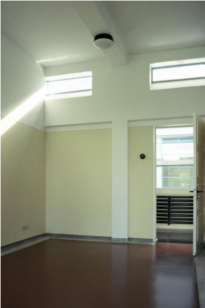
Sanatorium Zonnestraal, Hilversum (NL), archs. J. Duiker and B. Bijvoet, 1926-28, Main Building. Interior: bright light yellow walls with blue steel windows, brown linoleum in order to economize, photo: Mariël Polman, 2003
