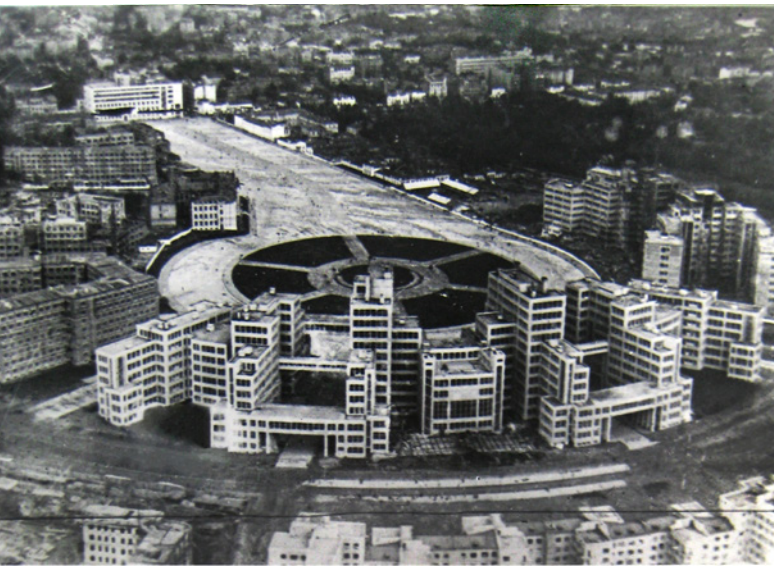
09 The ensemble of Dzerzhinsky Square during its creation. In the foreground: new residential high-rise buildings and Derzhprom; on the right—the House of Projects, on the left—the House of Cooperation, both in the process of construction. At the far end of the rectangular part of the square is the building of the Central Committee of the Communist Party of Ukraine; to its left is the building of the International Hotel under construction. © Unknown, photo of the early 1930s / [Photo of Dzerzhinsky Square]. Grigory Lebedev papers (Fund 1042, Inventory 1, Folder 1, p. 459), Central State Archive Museum of Literature and Arts of Ukraine (CSAMLA), Kyiv, Ukraine.
