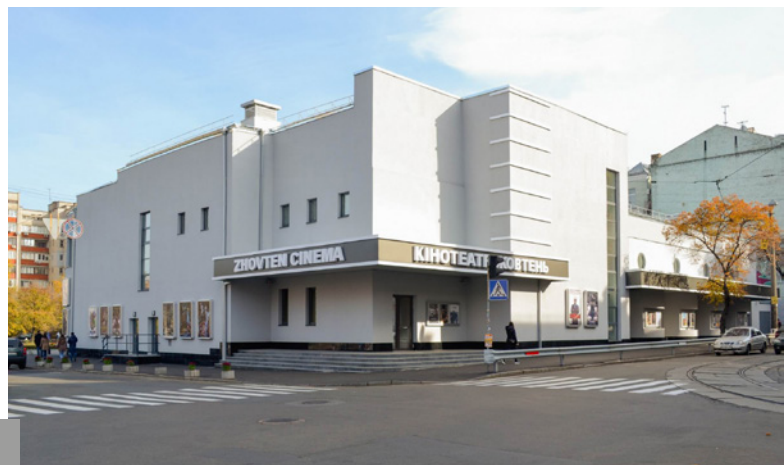
09 Kyiv, Kostyantynivska Street 26, "October" cinema. View after the last reconstruction with the reproduction of some original design elements. © https://kino-teatr.ua/uk/cinema-photos/jovten-16.phtml?photo_id=599 , 2017.
