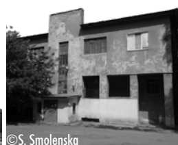
HOUSES FOR EMPLOYEES
