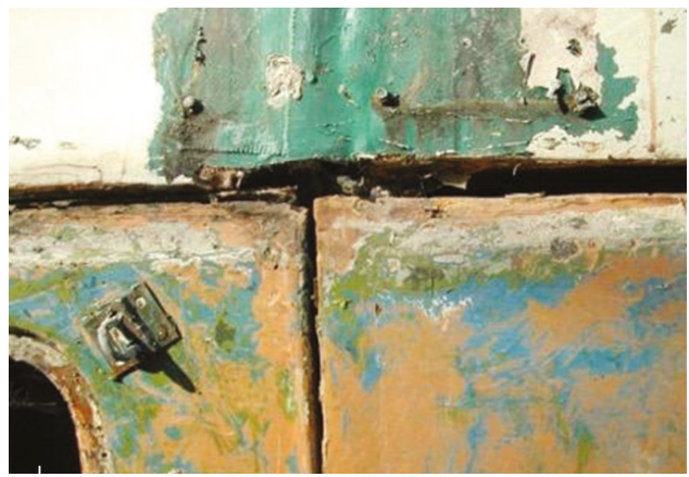
05 a-b One of the steel leg supports showing the typical extreme rust at the connection point (a) and (b) exterior of the Futuro near to top of the door opening where the top and bottom halves are joined. The vertical joint was where the two halves were connected with bolts. © M.W. Donaldson, December 2002
