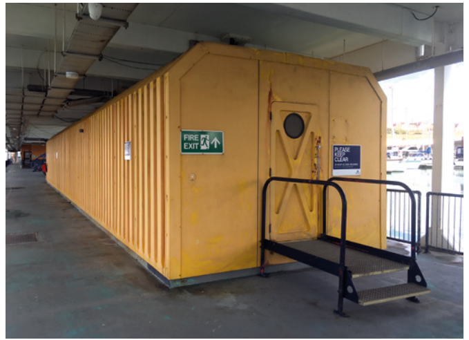
10 Building for Yachtsmen's Showers and Lavatories at Brighton Marina. © R. Loader, October 2019
