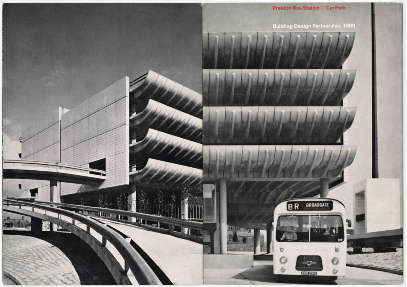
01 Keith Ingham for BDP, Central Bus Station and Car Park, Preston, Lancashire, England, 1969, west elevation as presented in printed publicity material. © BDP Archive (London), c1969
