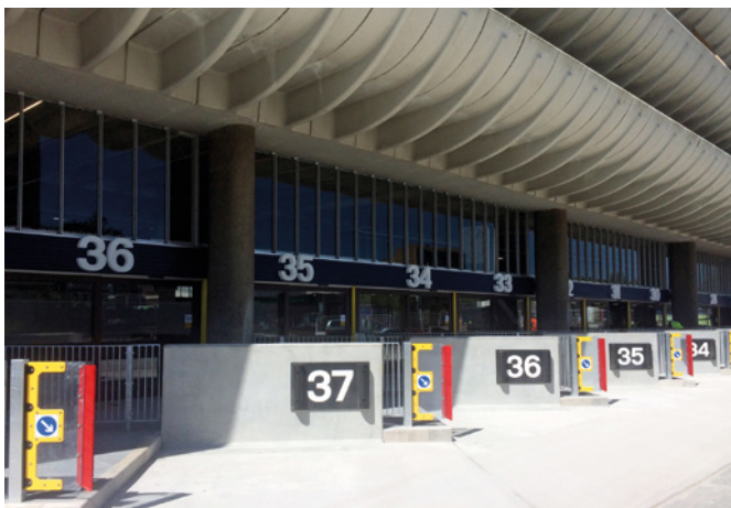
08 Keith Ingham for BDP, Central Bus Station and Car Park, Preston, Lancashire, England, 1969, bus station gates external signage, post-refurbishment. © J. Puttick, 2017
