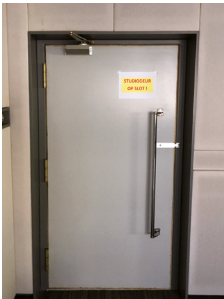
07 Door finished with synthetic fabric at the BRT Center. One of the few remaining witnesses of the initial presence of synthetic materials in the building. © N. Serneels
