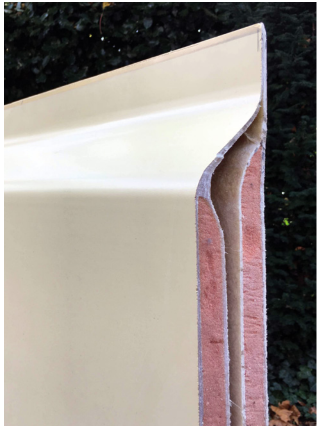
09 Cut-away section through a typical Herman Miller panel showing the double sandwich panels and air cavity. The panel face is painted, but the original gel-coat colour is visible around the perimeter edge. © R. Loader
