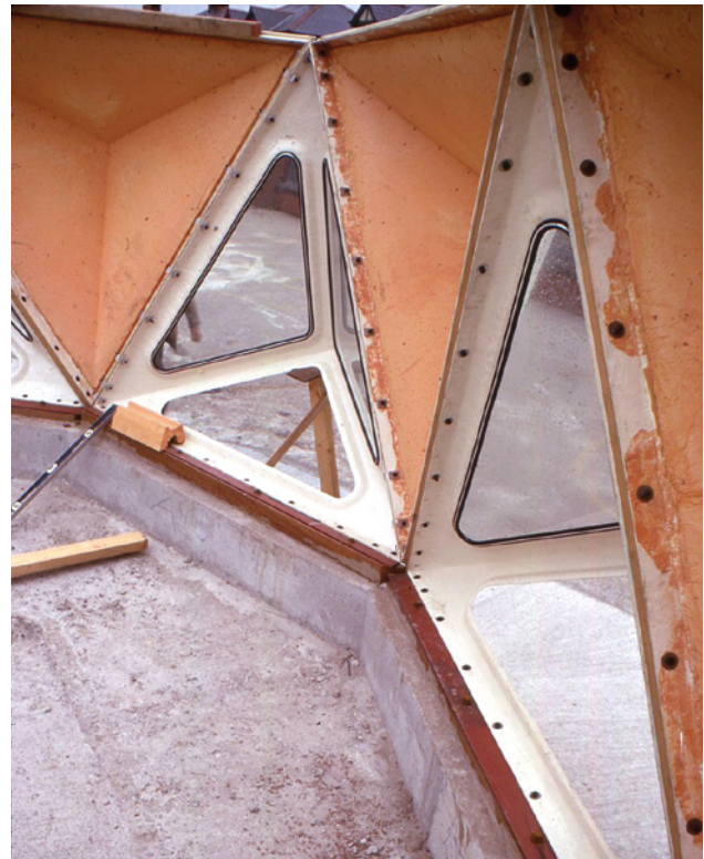
07 Photo during construction showing the pink exposed phenolic insulation (subsequently painted). The panel to panel joints are yet to be clad with pre-formed phenolic groins. © M. Bracewell
