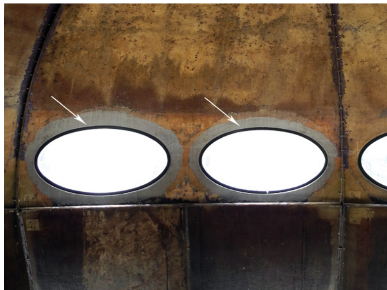
02 View of the interior depicting element 4T. The arrows point the newly reshaped openings. © E. Stamatopoulou, 2008
