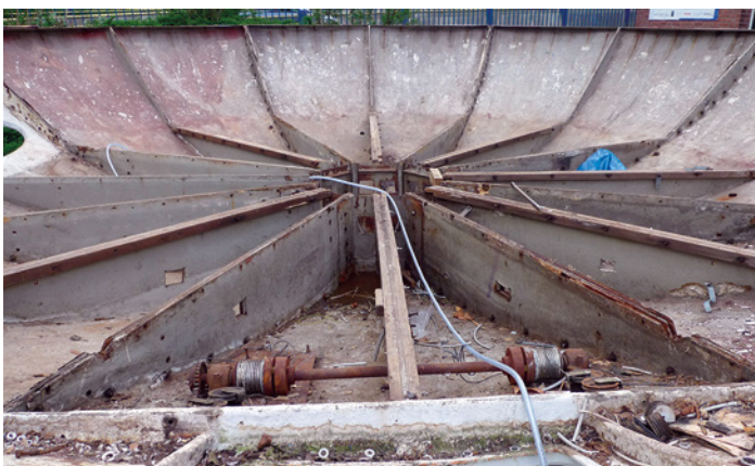
15 Support structure of the Finnish Futuro. © P. Voigt, 2016
