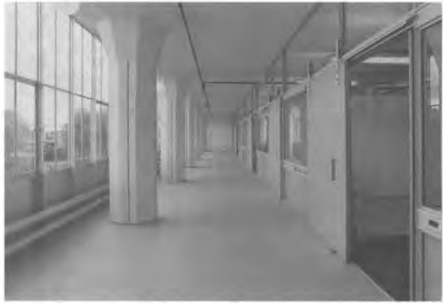
The secondary glazing at the shade side of the building is located at 2.25 m from the facade, creating a semi-climatised corridor. Note the spheric lamps. Photo: Fas Keuzekamp.
