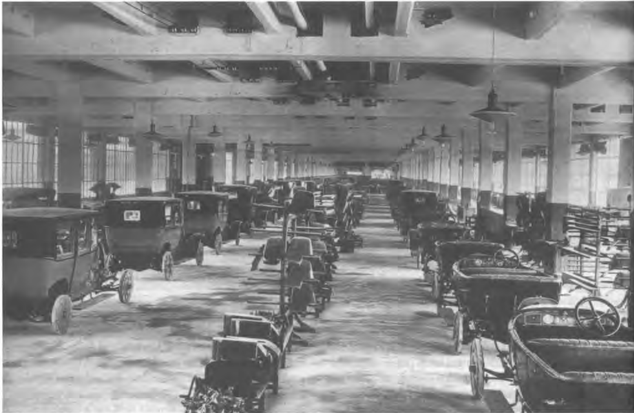
The original assembly lines at the New Workshops of the Lingotto complex in Turin. Note the floor beams with indents for the driving gears of the machines. Period photo from: Olmo, 1994.
