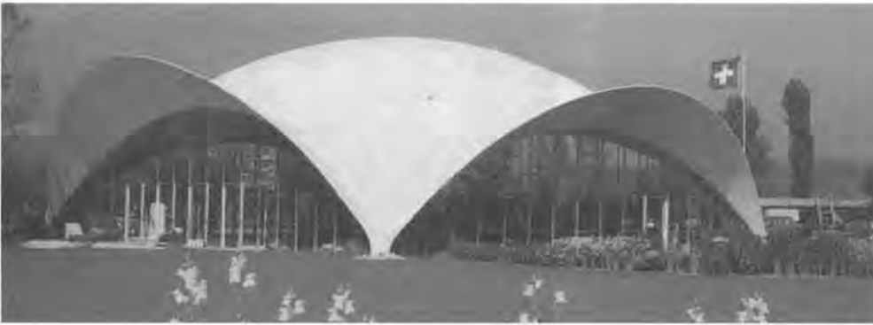
The free-form shell of the Wyss Garden Centre, designed by Heinz Isler 1962. Photo from the reviewed book.
