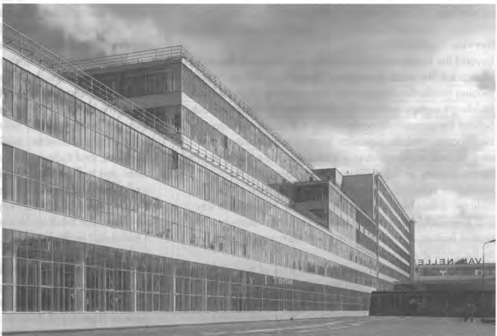
he visibility of the added secondary glazing depends on the weather conditions. At the this side, the new glazing is located just at 1.00 m from the original facade. Photo: Syboll Voeten architectuurfotografie.
