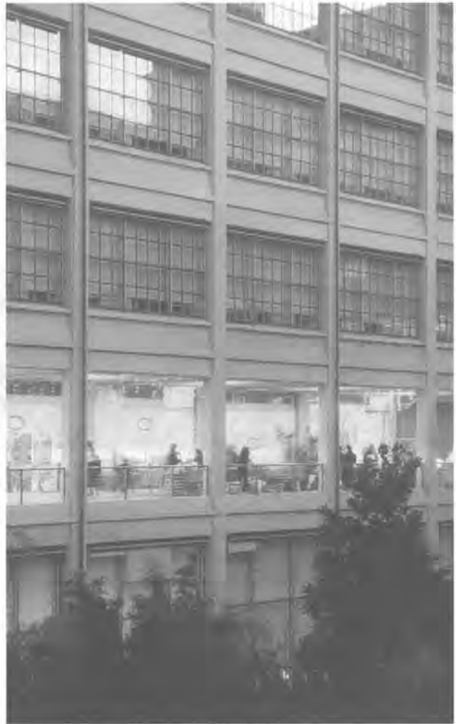
The shopping gallery has been cut out behind the concrete-framed facade and runs over the full length of the building. Photo: W. de Jonge.
