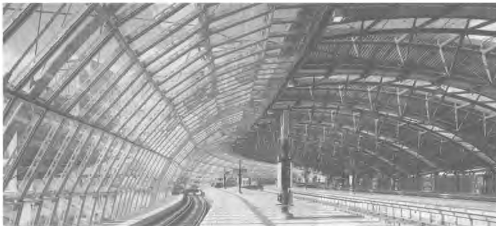
Waterloo International Railway Terminal, London, designed by Nicolas Grimshaw and Anthony Hunt in 1992. Photo from the reviewed book.
