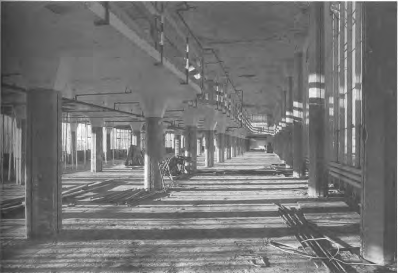
The empty space of the former coffee roasting department presented itself as a godsend, that will be used as a lunchroom with general services.
