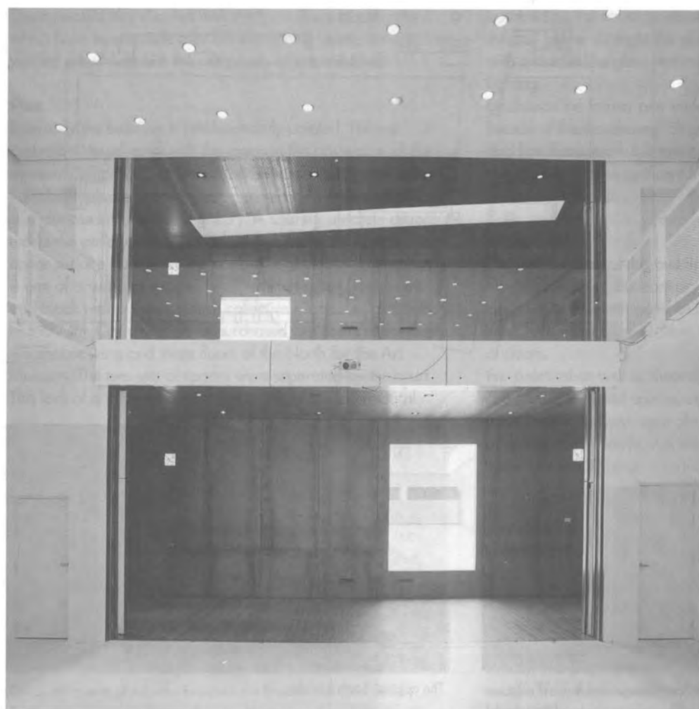
Top: The courtyard after Studio Granda's intervention. Two pairs of folding steel doors offer an array of opening possibilities to this multi-purpose space. Photo: Kristján Pétur Guðnason and Christopher Lund.
