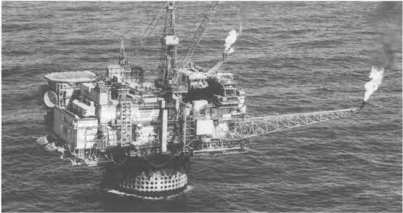
Ninian Central platform in operation, after removal of a redundant drilling rig and replacement by a new gas production module; 1991-1993. Photo courtesy of Chevron UK.
