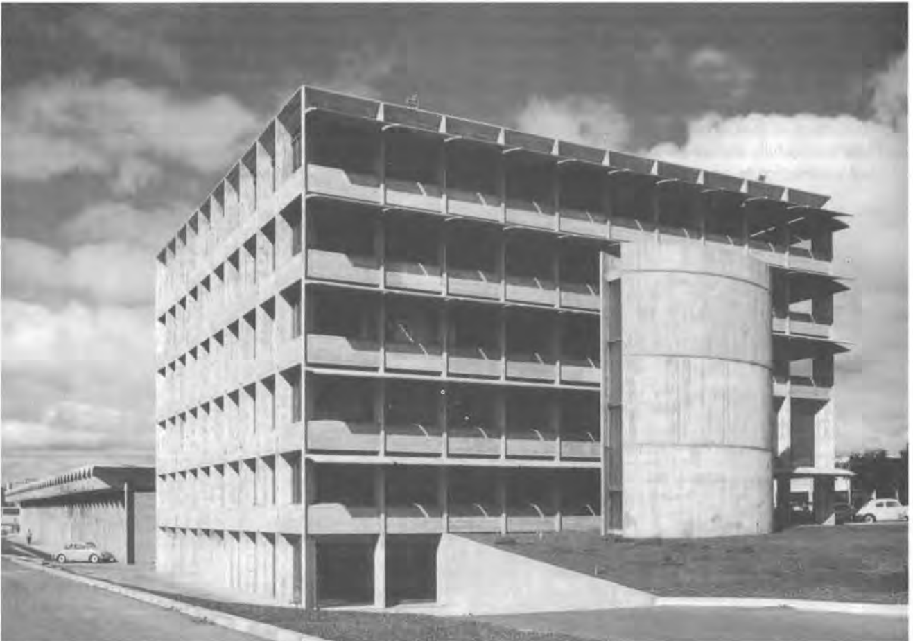
The Disbrave/Volkswagen plant in Brasília (1965) was one of Lelé's first experiments with prefabricated concrete. Photo from the reviewed book.
