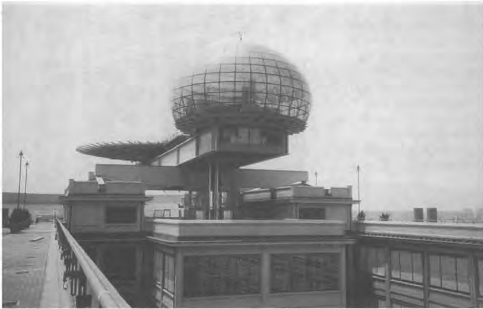
The spherical VIP-room, balanced by a helicopter platform; on one of the transversal blocks. Photo: W. de Jonge.
