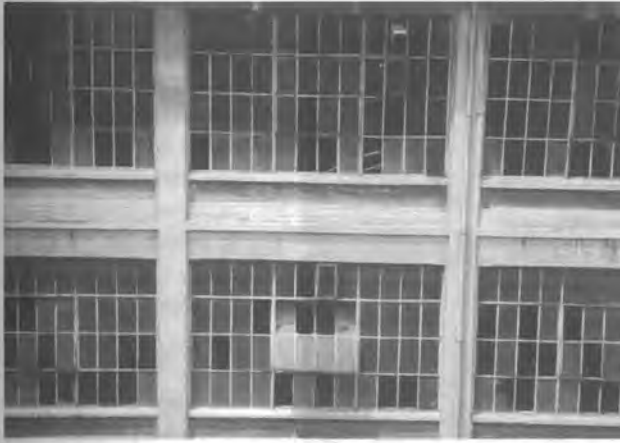
The original steel framed windows as found in the existing building, featuring 4x12 panels, were irreversibly lost. Photo: W. de Jonge.
