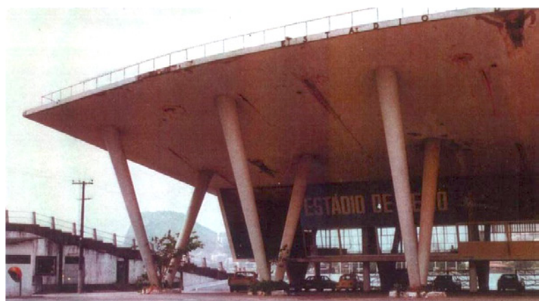
06 The lightness of the 1950s Block 1, with the V-shaped pillars elegantly supporting the grandstand, complemented by the subtlety of the pilotis and the translucent floors. © Available at http://urbecarioa.com.br/o-nao-legado-do-estadio-de-remo-da-lagoa-rodrigo-de-freitas/ . O "Não-Legado" do Estádio de Remo da Lagoa Rodrigo de Freitas. [Accessed April 23, 2021].
