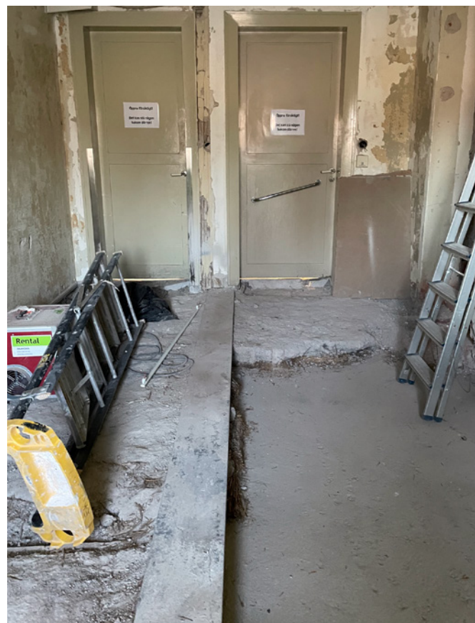
07 The local intervention and exposed layers of Solomite and aerated concrete materials in the library's uppermost floor in the 1932 western wing. © Marcelo Rovira Torres, 2022.
