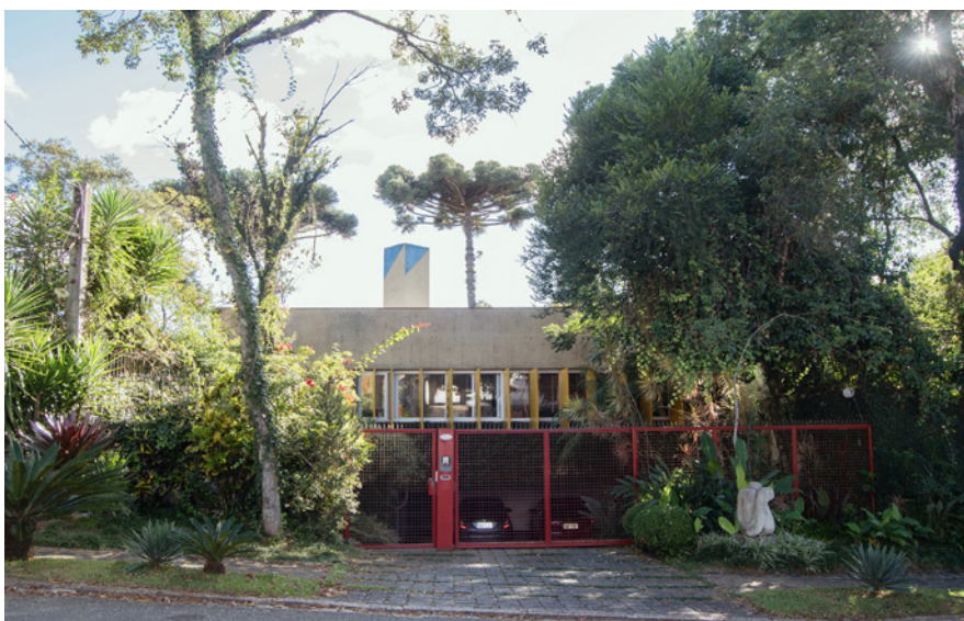
01 Manoel Coelho's house, front facade. © Author, 2022.
