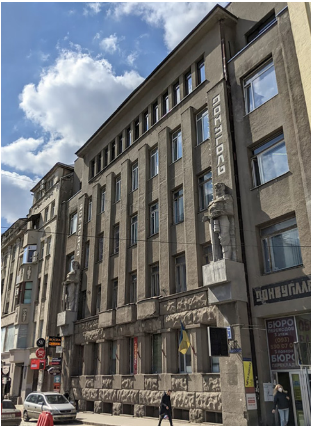
07 "Donugol" Trust on Pushkinskaya street, 5 in Kharkiv, 1925, architects A. I. Nossalevich, I. A. Lomaev, sculptor I. P. Kavaleridze. © O. Remizova, 2021.
