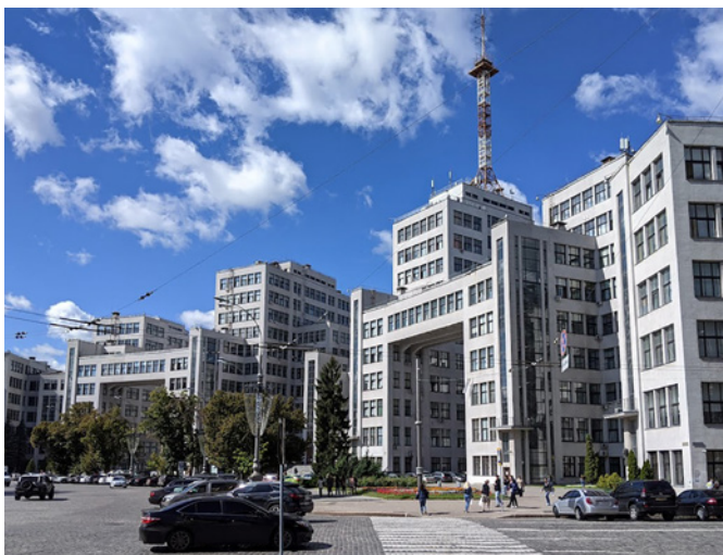
03 View of Derzhprom from Svobody Square in Kharkiv, architects S. S. Serafimov, S. M. Kravets, M. D. Felger. © O. Remizova, 2021.
