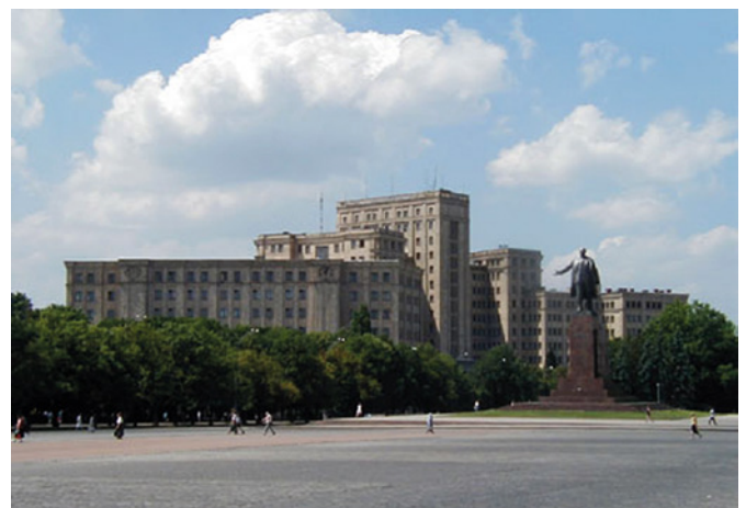
09 V.P. Kostenko, V.I. Lifshits and others. The main building of V.N. Karazin Kharkiv National University (KhNU) (Reconstruction of the former House of Projects). Kharkiv. Ukraine. 1953—63. © Ryzen, 2008. https://commons.wikimedia.org/wiki/File:Place_de_la_libert%C3%A9.jpg .
