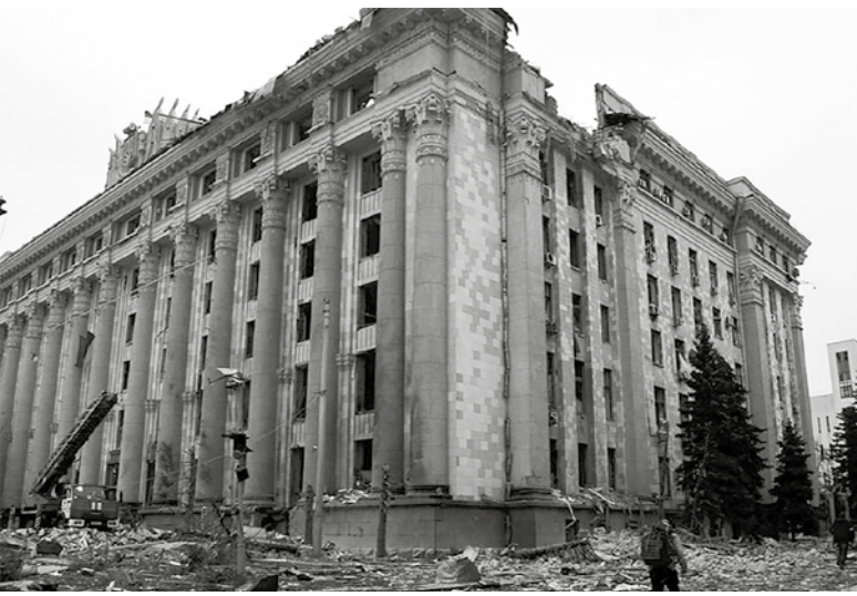
02 The building of the Kharkiv Regional State Administration after the bombing. © Andrey Maiaenko, UNIAN: News of Ukraine, 2022.
