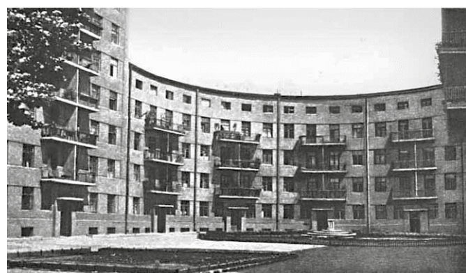
07 Komunar (Communard) residential house, 1929-1930, arch. A. V. Linetskiy and V. I. Bogomolov. © prof. A. Bouryak's personal archives.
