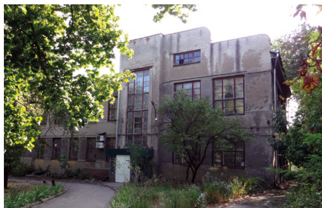
11 UPhTI. The laboratory building. © Photo by S. Smolenska, 2020.
