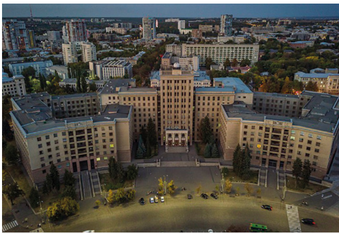
10 P.E. Shpara, N.P. Evtushenko and others. Northern building of KhNU (Reconstruction of the former House of Cooperation). Kharkiv. Ukraine. 1954. © K. Brizhnychenko, 2020. https://commons.wikimedia.org/wiki/File:Будинок_кооперації,_Харків_DJI_0050.jpg .
