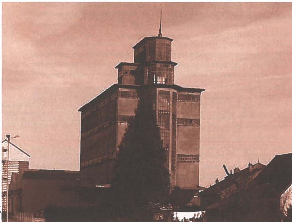
Fig. 1. General view of building
