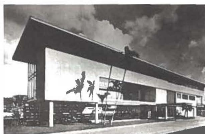
fig.2 Mario Romanach: House Noval Cueto, La Habana, 1949. Main façade.
