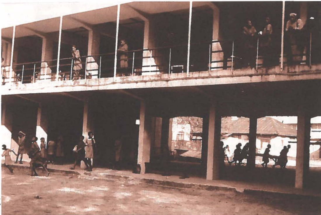
Fig 2 . Godwin and Hopwood, Christ Church Cathedral School, Lagos, c. 1957. Classroom layout and "pilotis" ground floor structure.
