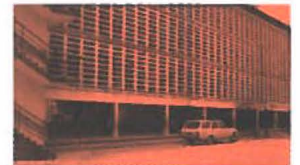
Fig. 3. Godwin and Hopwood, Anglican Girls Seminary School, Lagos, c. 1957. Extensive use of shading devices.
