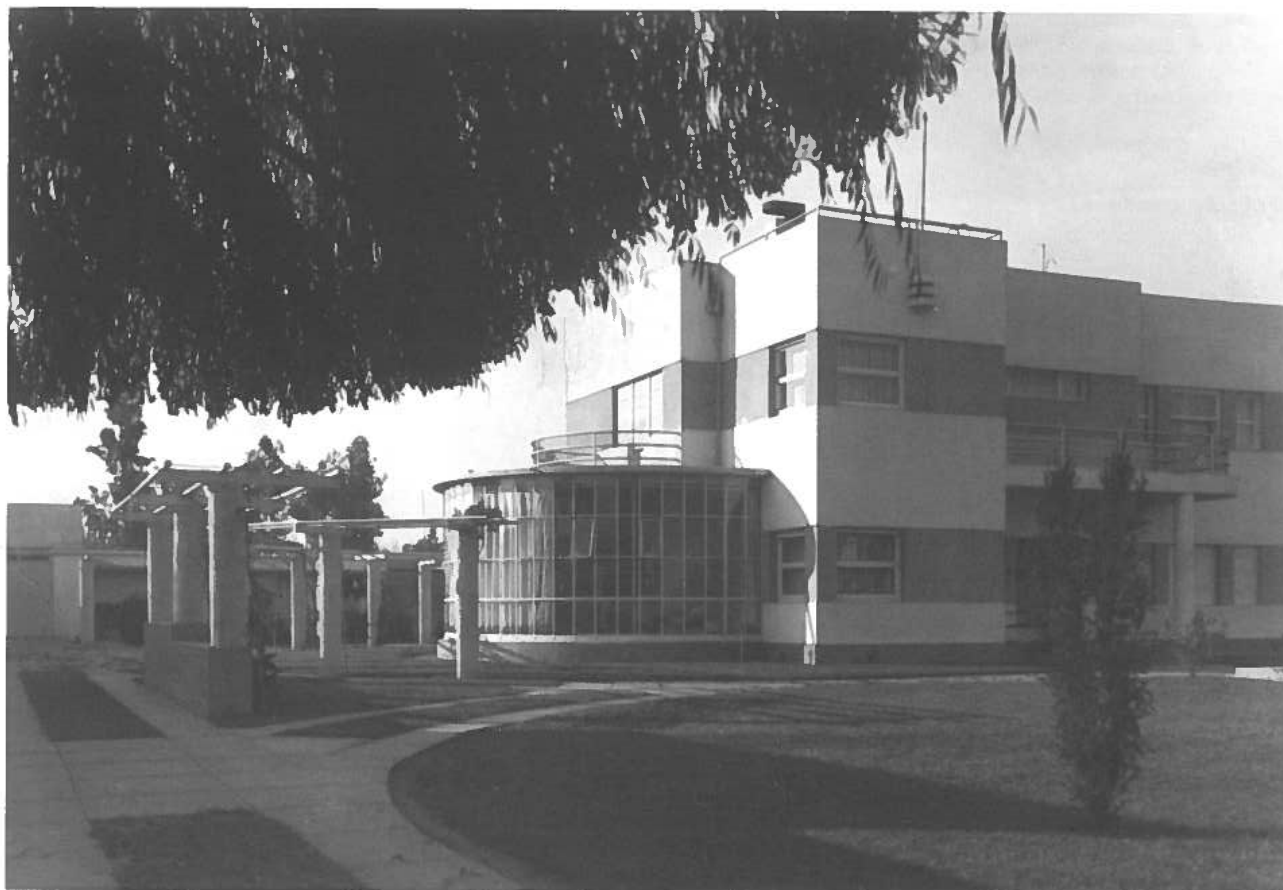
Fig. 2. Fedorov y Hayme , the Hasbun House, detail of the South-western corner, Santiago, built in 1935. Demolished in 2004
