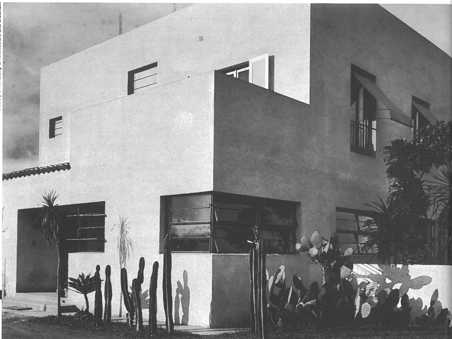
Gregori Warchavchik , architect's residence, São Paulo, 1927–28
