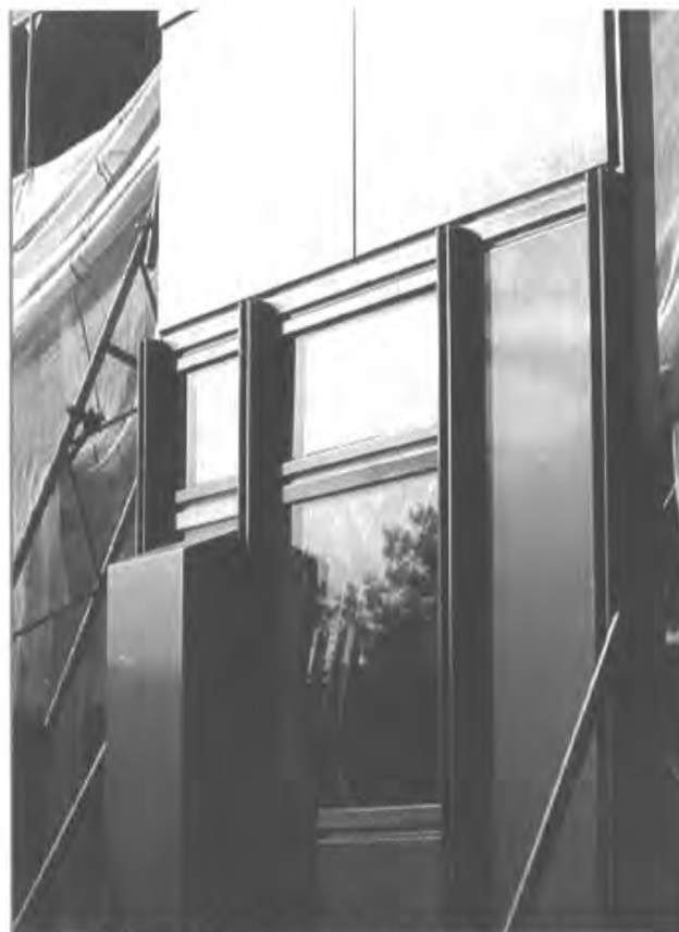
Mock-up of the replacement facade in bronze, designed by Foster & Partners. Photo: Foster & Partners, Berlin.
