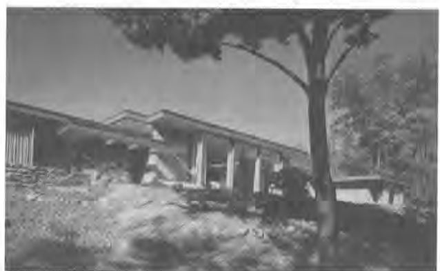
Gores House, Landis Gores, 1948. In this house, one of the early Harvard Five houses, Gores combined glass, field stone, vertical wood siding and large overhangs to visually anchor the house to the landscape and emphasize its horizontal lines. Gores later designed a series of stepped terraces and a pool level to replace the natural slope seen in the foreground of this early photo. Photo: Courtesy Pamela Gores.
