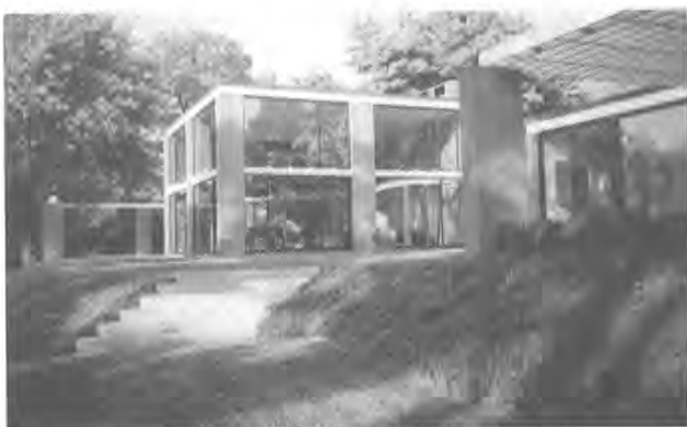
Boissonas House, Philip Johnson, 1956. Johnson's Boissonas house followed his Glass House by several years, but utilized brick and glass to similar effect in a more complex and expansive scheme. The double-height living/dining room is flanked by two lower wings with glass walls on the garden/pool elevation and more conventional, less transparent walls on the entry elevation. Photo: Robert Thomas.
