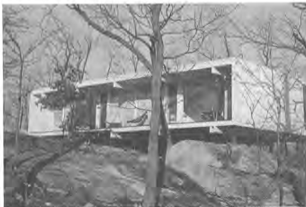
Lee House No. 1, John Black Lee, 1952. To preserve the natural qualities of the site, Lee designed this house to hover above a massive rock outcropping on 6 x 6 inch stilts. The rock drops off on the far side of the house providing the cantilevered bedrooms with tree-top views of the valley and meadow below. Photo: John Black Lee.
