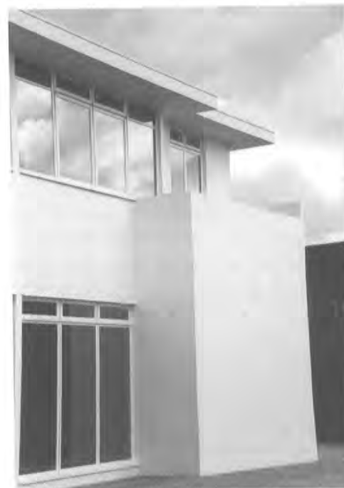
Detail of the house after restoration. Photo: Dennis Sharp Architects.
