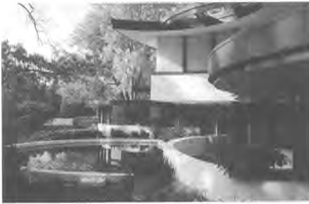
Leuthold House, Alan Gelbin, 1964-1966. Gelbin was a Taliesin Fellow and apprentice to Frank Lloyd Wright between 1949 and 1953. After serving as supervising architect for many of Wright's houses, including 'Rayward' the only house Wright designed in New Canaan, Gelbin designed houses on his own in the New England area. The Leuthold house combines stucco finished exterior walls with fascia and window framing of varnished mahogany. Photo: Robert Thomas.
