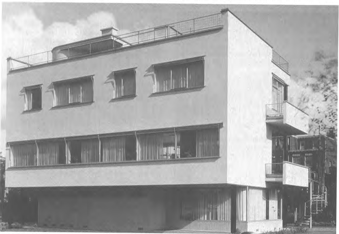
Period photo of the west elevation of the Sonneveld House, 1933. Photo: Jan Kamman, by courtesy of Van den Broek and Bakema archive/ Nederlands Foto Archief.
