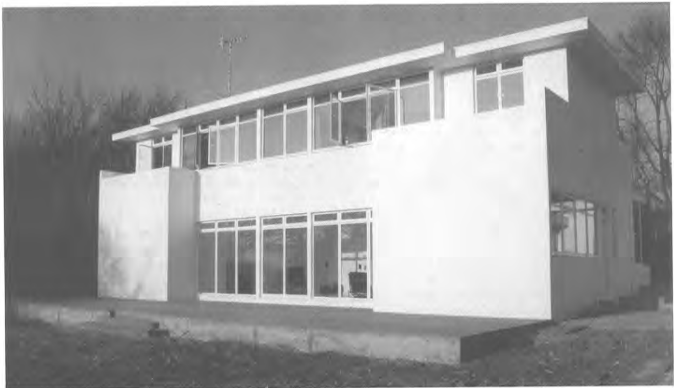
Garden elevation of the house after restoration. Photo: Dennis Sharp architects.
