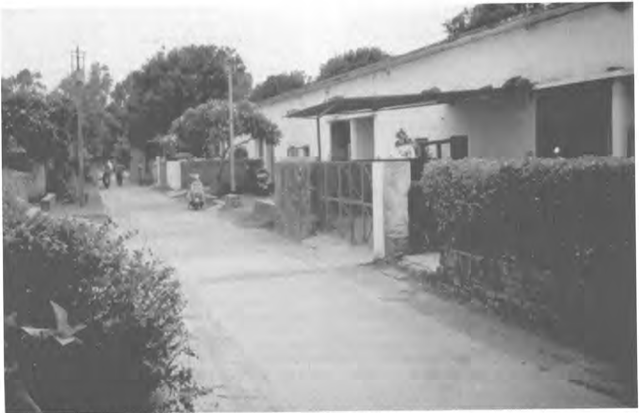
House type 13, designed by Jane Drew for sector 22. Forecourts are partitioned into individual plots and often accommodate parking sheds.
