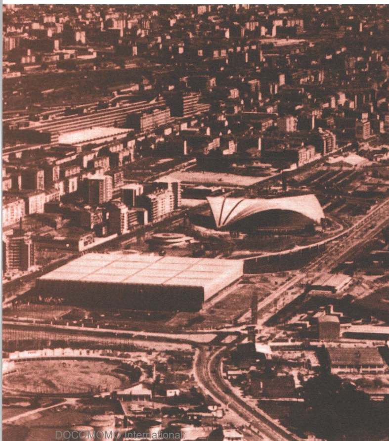
Fig. 8. Pier Luigi Nervi , aerial view of the Palazzo del Lavoro for the celebrations of Italia'61 for the centennial of the national unity, 1960
