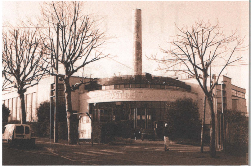
Entrance of the old incineration plant : the swimming pool occupied the left part of the building and the incinerator the right-hand side
