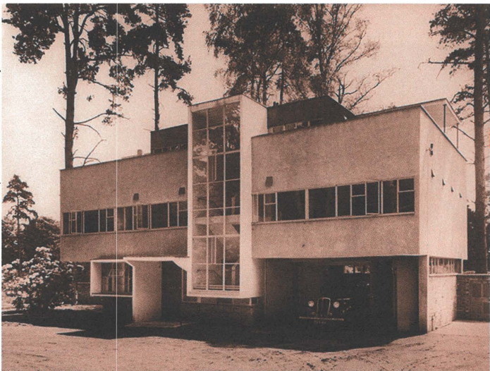
Photos: © Book Art Architecture Picture Library / Connell Ward & Lucas Connell Ward & Lucas , front façade of Greenside house (formerly Bracken), built 1933-39
