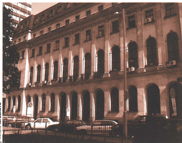
Asen Michailovski, Reconstruction and renovation of the Central Post Chamber, 1938
