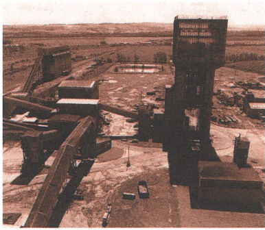
Fig. 1. Monktonhall Colliery. 1989 view from n°2 winding tower towards up-cast shaft, showing boiler house in foreground, conveyors to coal preparation plant and rapid loading bunker
