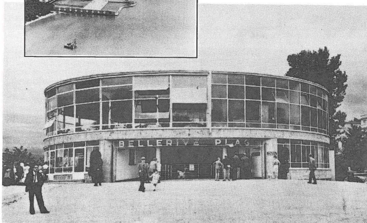
Left: aerial view of the Bellerive Baths on a period photo, around 1937. Bottom: the rotunda and the entrance in the late 1930's. Photos: Musée Historique de Lausanne.
