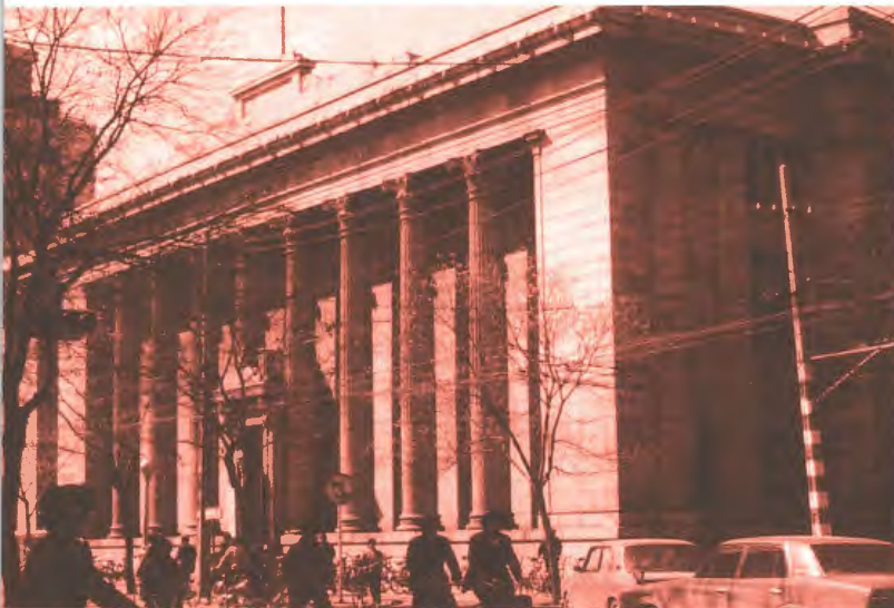
Fig. 4. Atkinson & Dallas (attributed), Yokohama Specie Bank , now the China Bank, 80 Jiefang Bei Road, 1925-26
