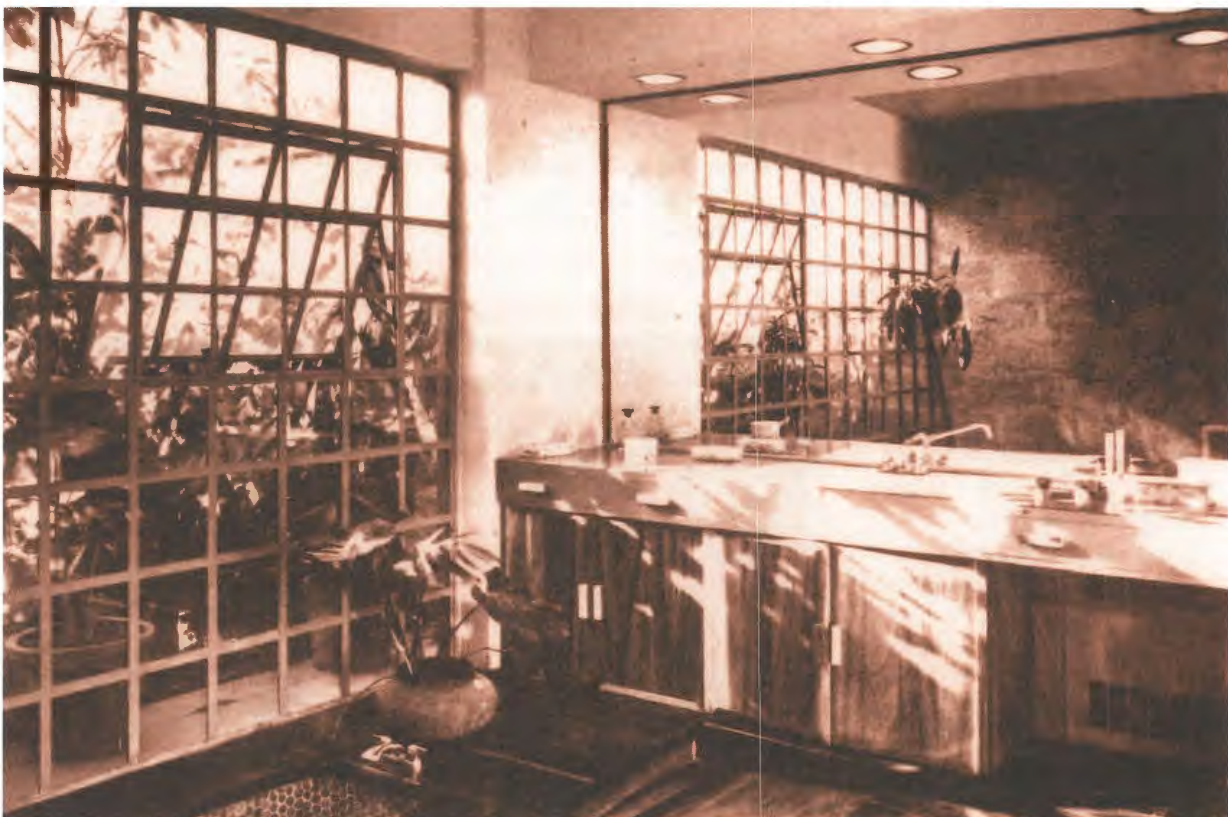
Fig. 1. View of the bathroom
