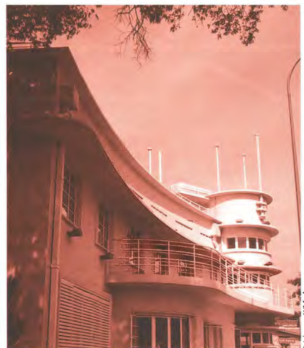
Fig. 7. The Waterboat office by Swan & Maclaren (1919). Today, the renovated building is a restaurant
