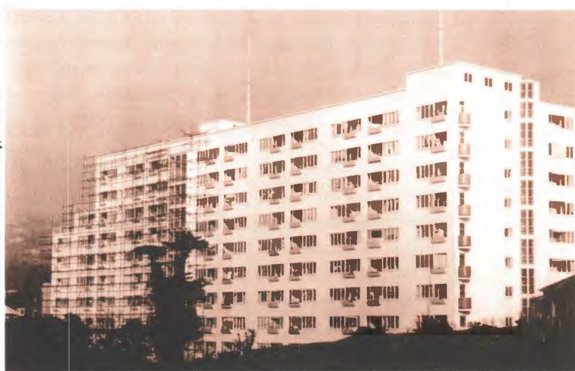
Fig. 3. Department of Housing Construction, Dixon Street Flats, Wellington, 1942
