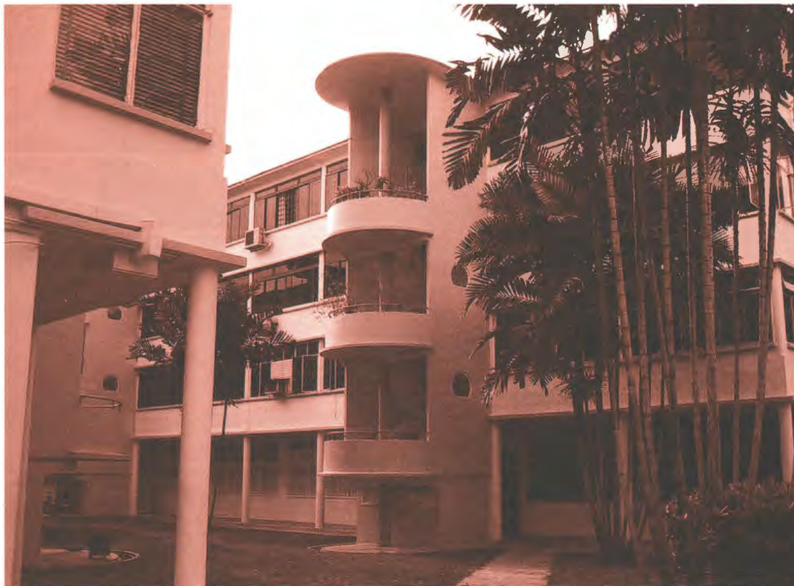
Fig. 3. Low-rise SIT apartment building in Tiong Bahru
