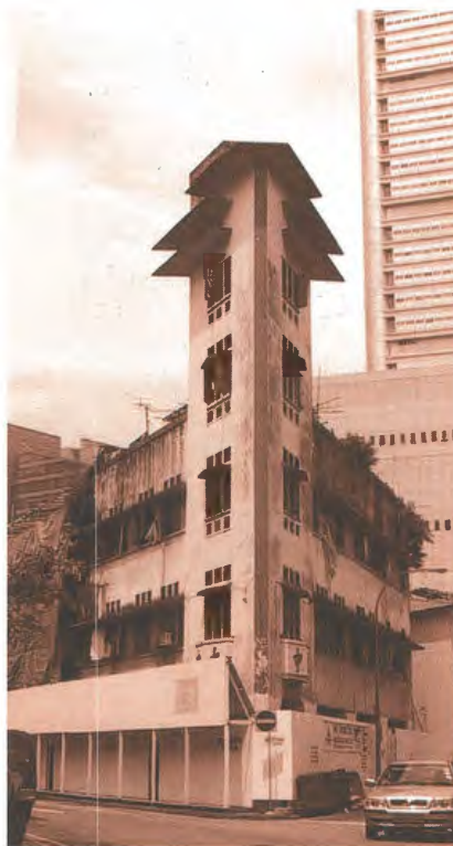
Fig. 8. A corner building by Ho Kwong Yew, in the Raffles Place area, in its recent state of dilapidation and now in the process of being renovated
