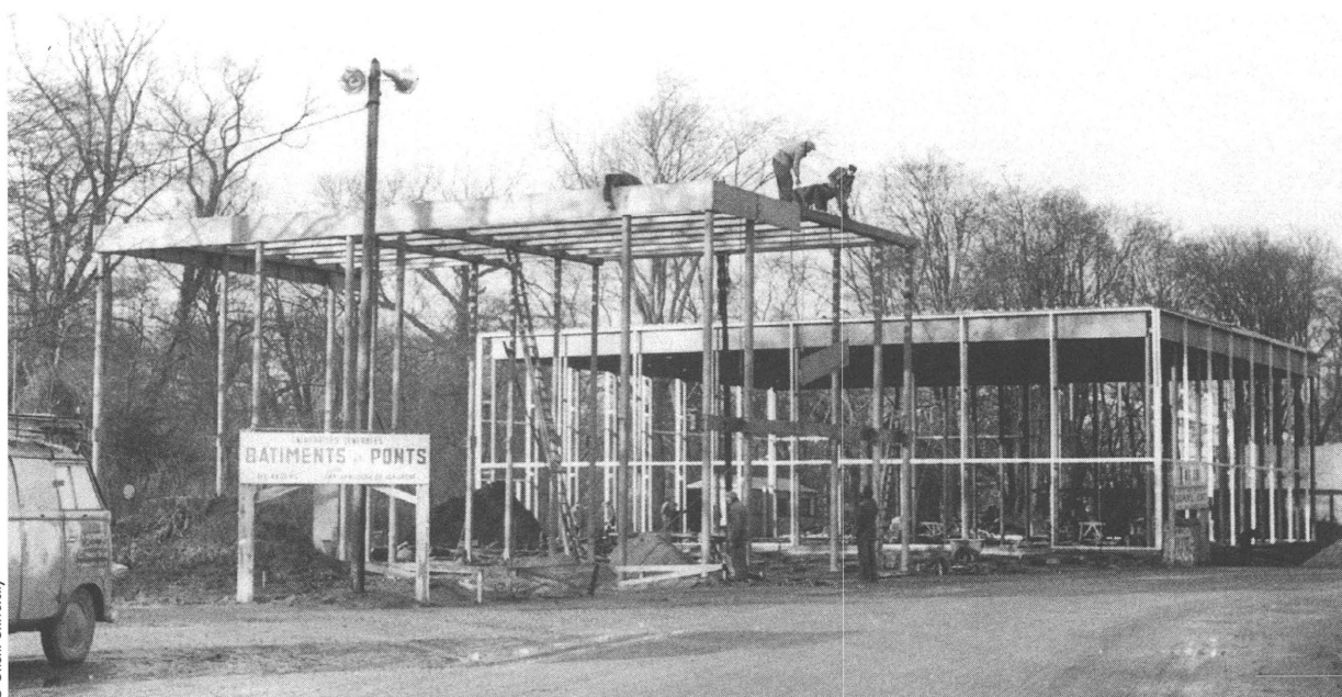
Fig. 2. Construction photograph of the Pavilion showing the modular steel-frame structure
