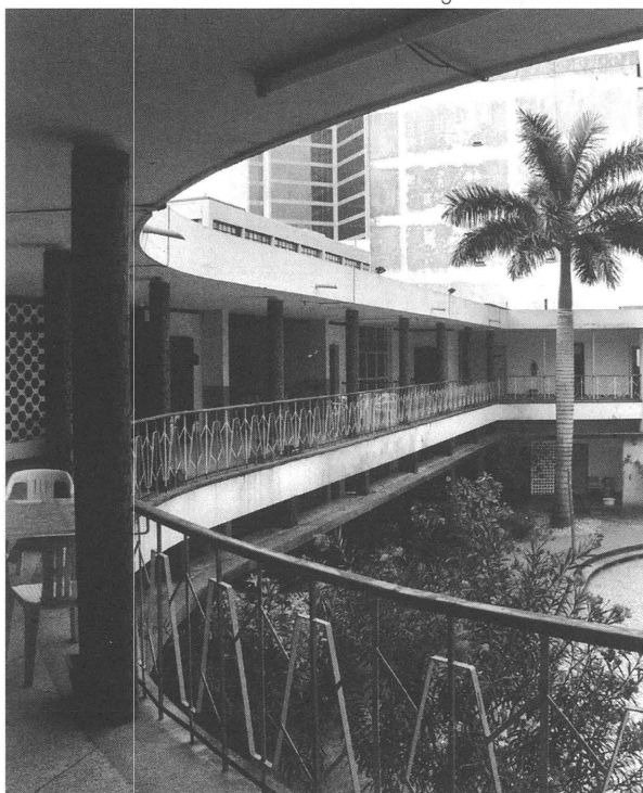
Anthony Almeida , Goan Club , looking over internal balconies
