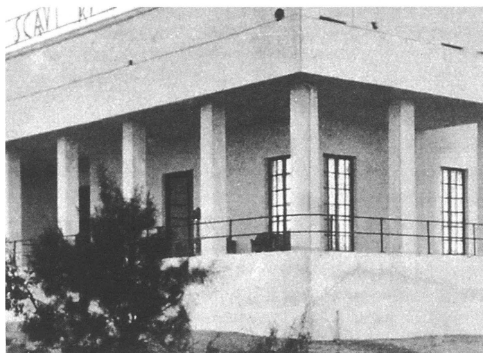
Fig. 4. The Hotel at the Leptis Magna Ruins. Front façade, detail of the colonnaded veranda
