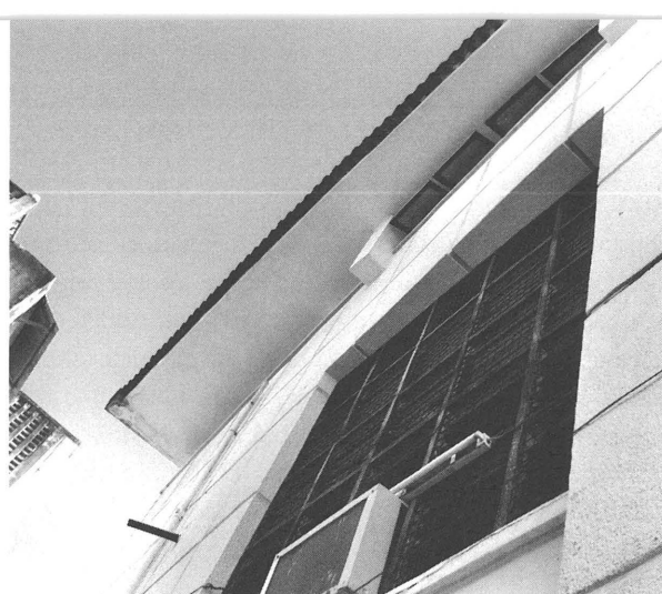
Amyas Connell, detail of the elevation of the Novelty Talkies picture house, Tanga, c. 1949
