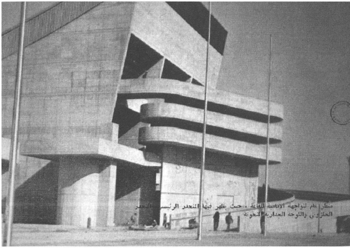
Fig. 2. Le Corbusier's Baghdad Gymnasium building. When the gymnasium opened in 1980, this photo featured on a propaganda booklet highlighting the design features of the newly named Saddam Hussein Gymnasium
