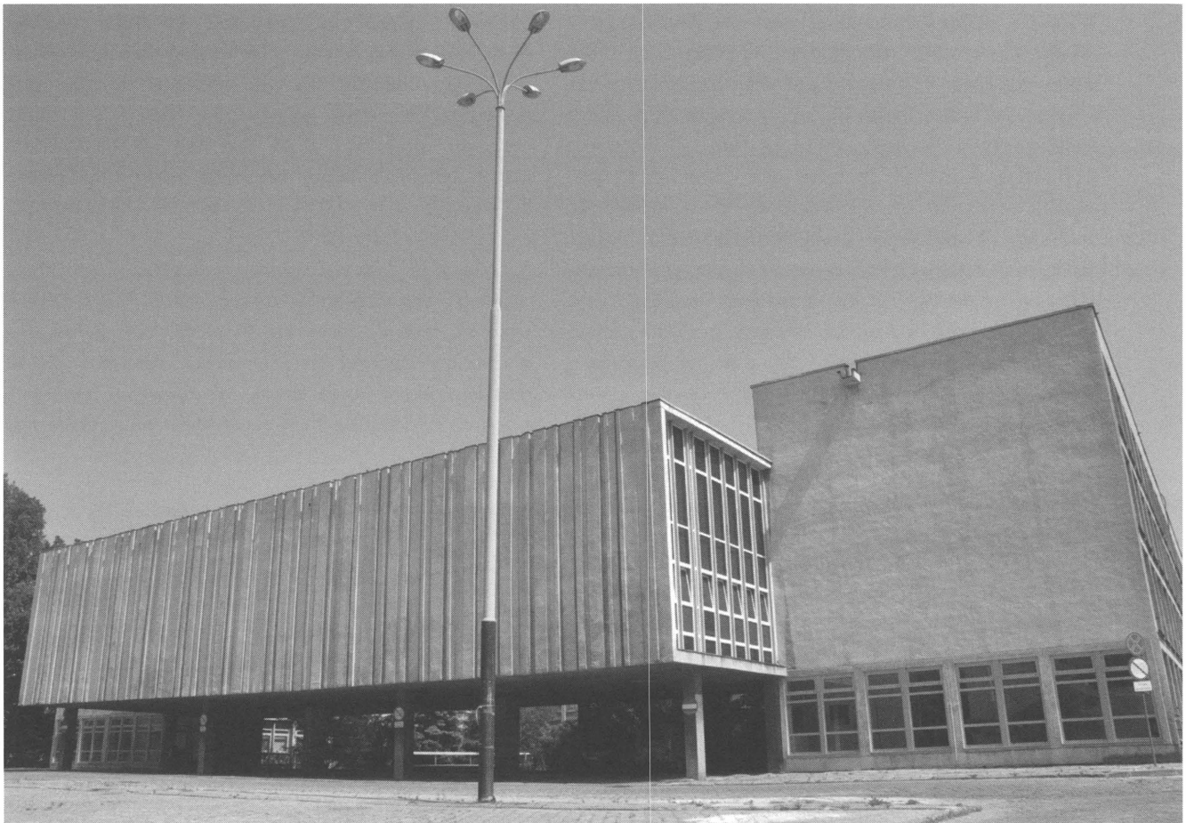
Fig. 1. Boleslaw Kardaszewski, Ludwik Mackiewicz , Building Center of Technical University of Lodz, Lodz, 1969–1975
