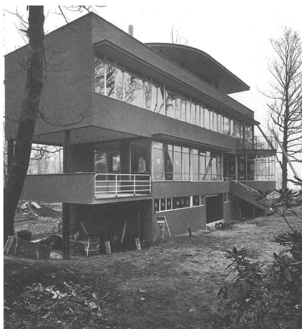
Fig. 7. Basil Ward's house at Moor Park of 1936–1937 was next to a golf course in a private road. It is one of the most radical of all the houses of the decade using a system of reinforced concrete post and beam construction
