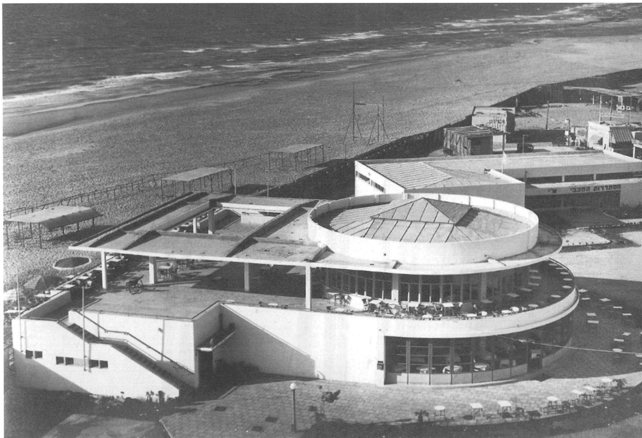
Fig. 3. Averbuch & Ginzburg, Gidoni , Galina Restaurant , one of the most outstanding pavilions in the fairgrounds, 1934. Destroyed
