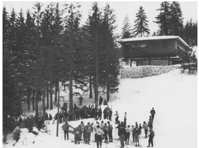
03 Juraj Neidhardt, The ski house on the Trebević Hill near Sarajevo, 1947-48. © Tatjana Neidhardt.
