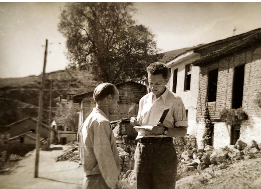
01 The team taking site notes somewhere in Macedonia, 1947-49. © Grabrijan and team, Grabrijan archives, Folder 4, drawer 5.2: Macedonian House, Museum of Architecture and Design, Ljubljana.
