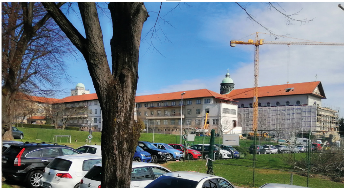
06 Renovation after the 2020 earthquake in 2023. © Darja Radović Mahečić, 2023.
