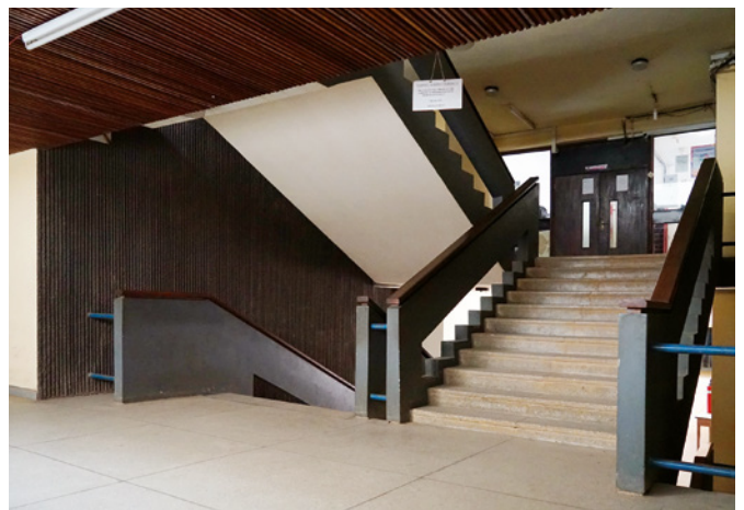
18 Obafemi Awolowo University, Library, circulation area with terrazzo flooring, raked spray render wall surfaces, wooden ceiling cladding and handrails, painted concrete, blue metal railings, 2022. © Brenne Architekten, 2022.
