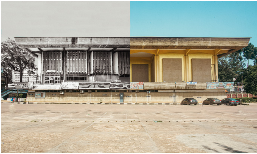
34 Synthesized picture of the main library and main auditorium, showing the similarities in structure and external finishes of both buildings. © Bola Oguntade, 2022.
