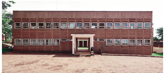
25 Main entrance of the Faculty of Education designed by Peatfield and Bodgener in 1988, Kyambogo University, Kampala, Uganda. © Timothy Latim, 2022.
