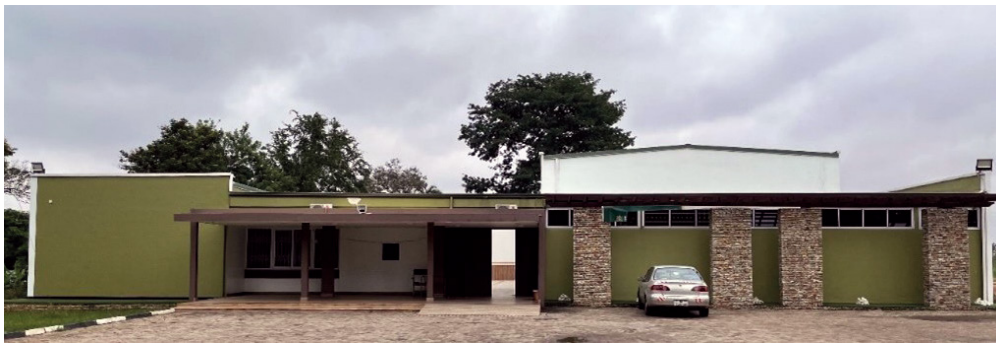
06 KCC after renovation, front view towards entrance and view of open court. © Author, 2023.
