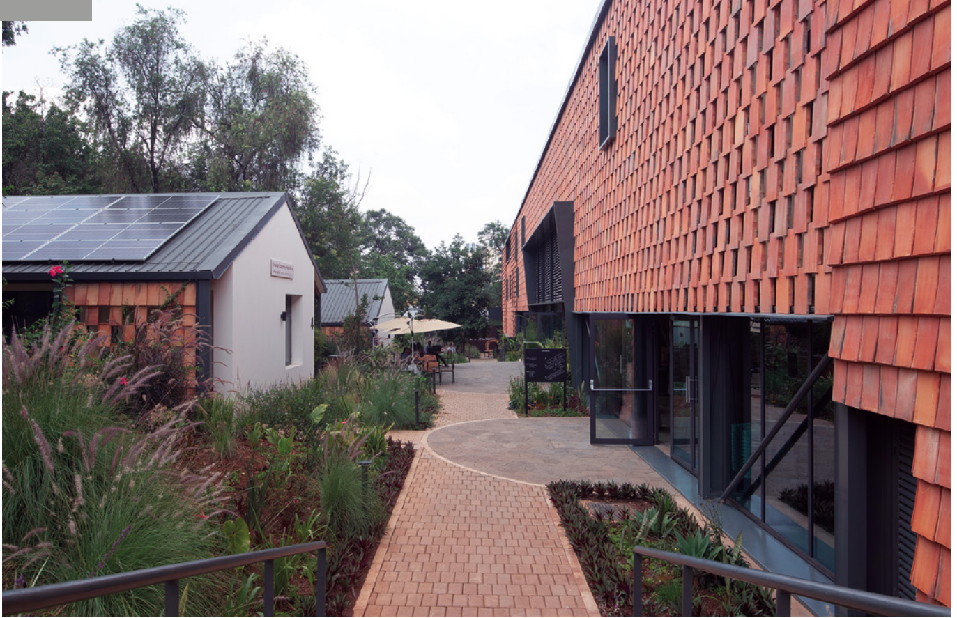
04 The main Norrskén House and refurbished classroom blocks designed by MASS Design Group. © Author, 2023
