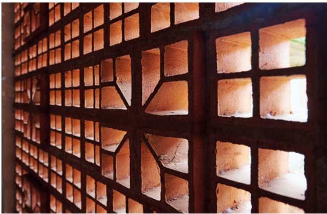
07 Detail of the hollow blocks at the east and west facades of Rukurato Hall. © Timothy Latim, 2023.
