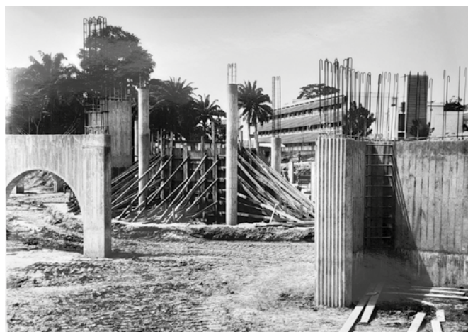
03 University of Ife, Assembly Hall, corrugated reinforced concrete column under construction, November 5, 1973. © Israel Kainy.
