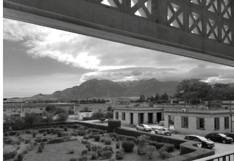
02 The School of Agriculture of Sidi Naceur in Mograne before the mountains of Zaghuan, seen from the entrance block. © Author, 2023.
