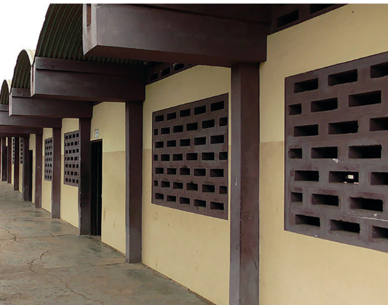
07 Veranda for circulation and roof overhangs for solar shading © Futurestars Charity, 2018
