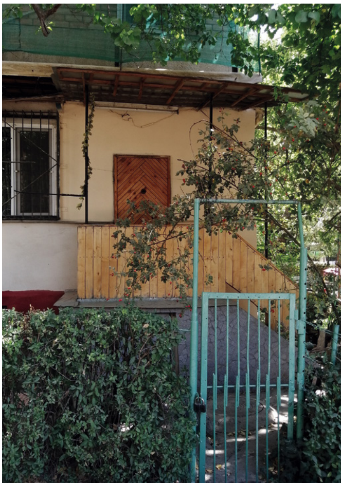
08 Self-adaptation of the ground floor of one of the Soviet housing series with the organization of a separate entrance to the apartment, taking over part of the adjacent communal territory, and rearrangement of the balcony. (Tashkent, YunusAbad -14). © E. Gladkova, 2022.
