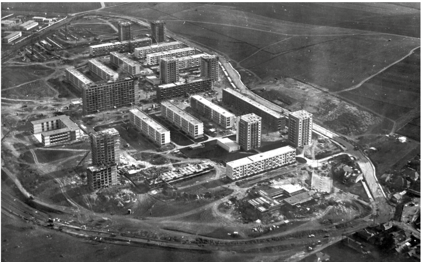
02 Gheorgheni housing estate, Cluj, microraison 1 in construction. © N. Kulin, 1965, DSAPC Cluj.
