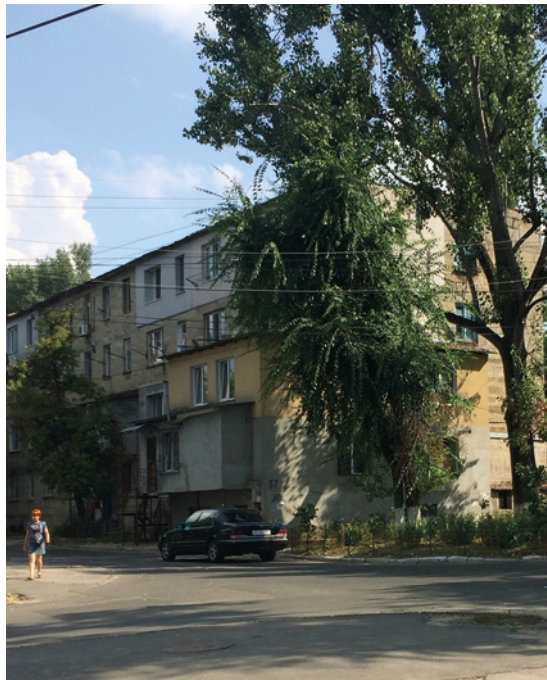
06 Self-alteration of the facade of residential buildings in Chisinau, Ion Neculce street (left), Mihai Eminescu street (right). © M. Sapunova, 2017.
