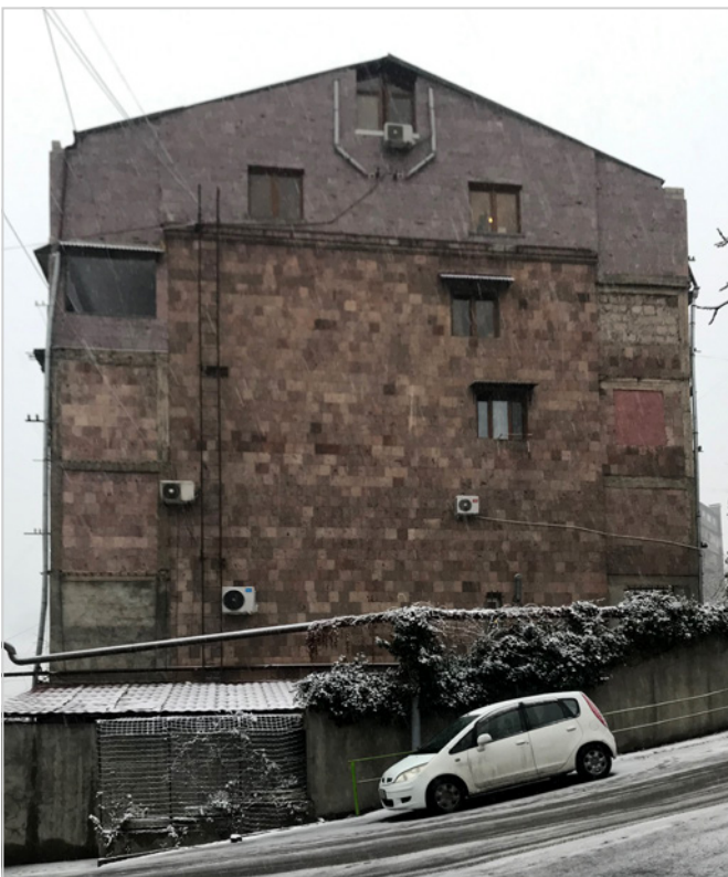
05 5-story apartment block with additional windows, additional balconies, and an upper floor in the central district of Yerevan, Saryan street. © M. Sapunova, 2023.
