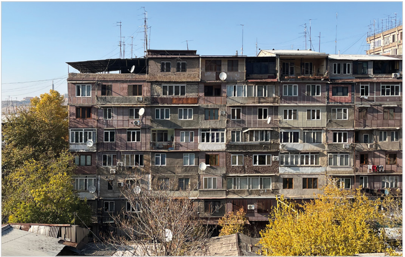
04 A mass residential building in Yerevan with an added top floor and individually glazed balconies. © M. Karaselnikova, 2022.
