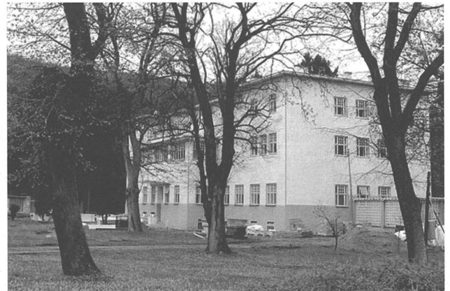
2.2. Purkersdorf Sanatorium in Lower Austria, architect: Josef Hoffmann, 1905. Photo: A. Huber.
