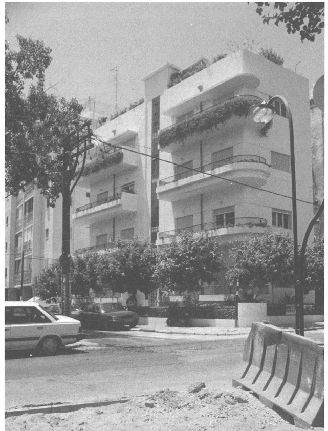
An apartment building at 32 Ben Gurion Boulevard, restored in 1998 adding a new floor by the architect Aharony. Photo: Nitza Szmuk.
