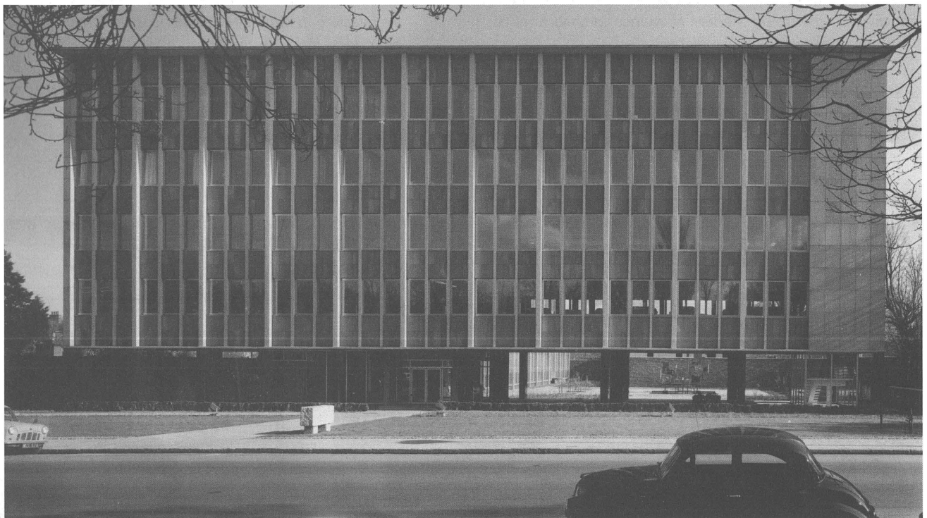
Pelican House, originally Irish Life Headquarters, Dublin (1959-63), designed by Downes, Meehan and Robson Architects, demolished 2001, front. Photo: Henk Snoek, 1964.
