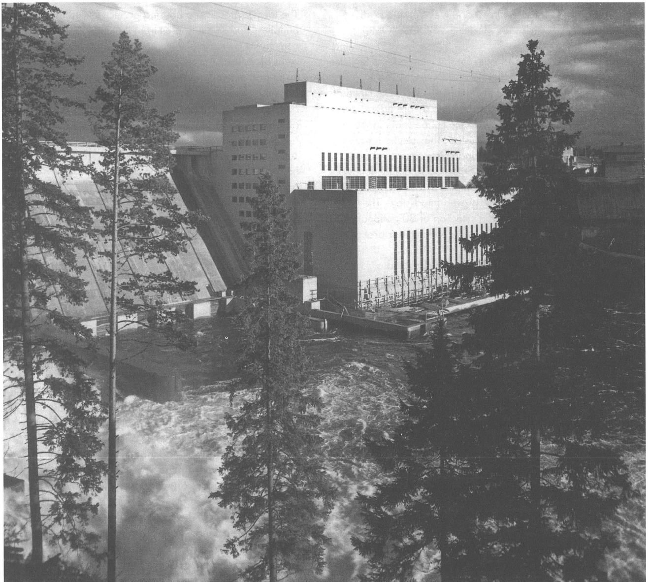
The Oulujoki power plant, designed by Aarne Ervi in 1947, is located in Pyhäkoski. Today, these plants are automated and the communities around them become obsolete. Photo: Roos, courtesy Museum of Finnish Architecture.
