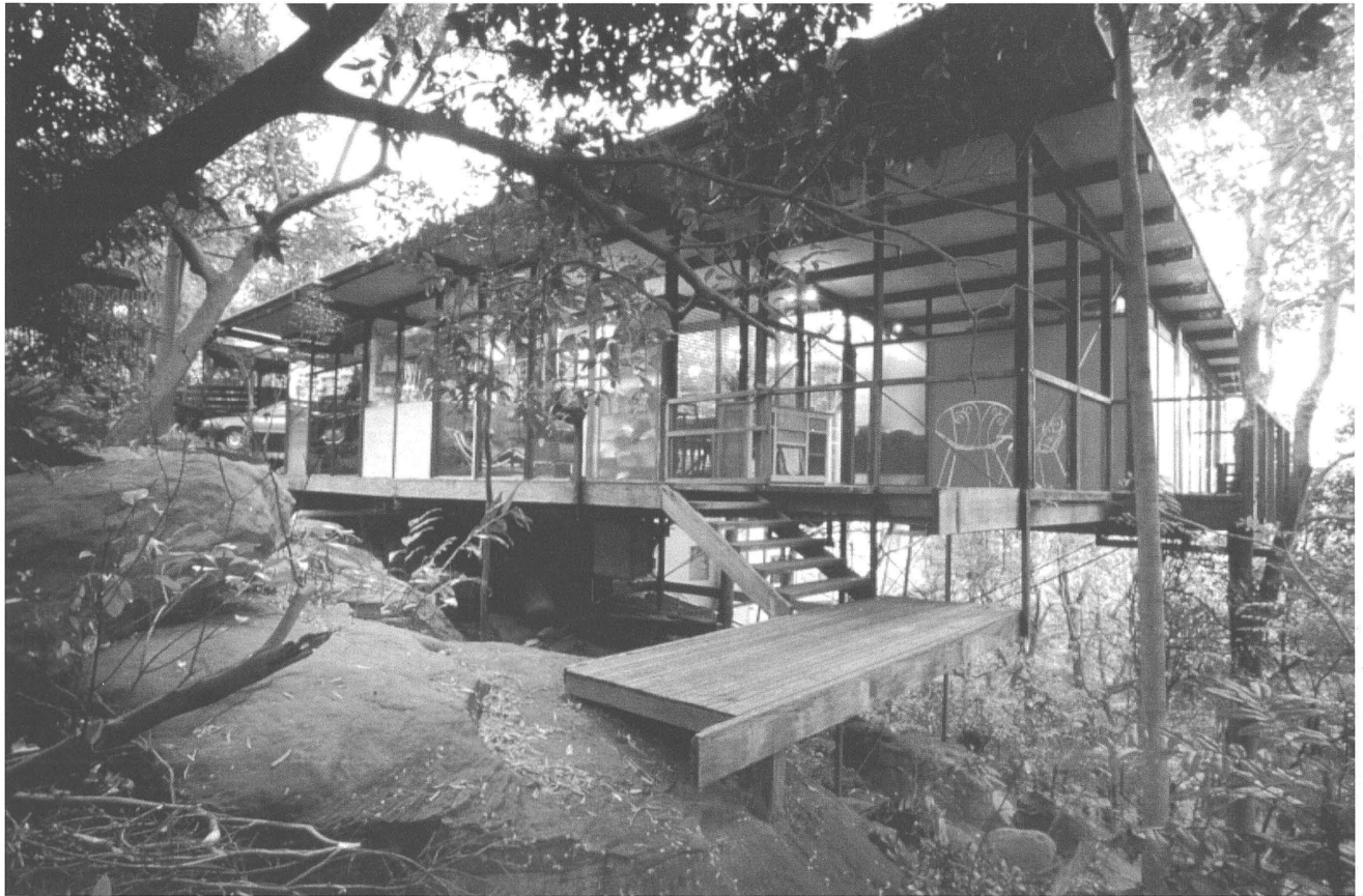
The Lucas House, Castlecrag, Sydney NSW, 1957. One of the six houses featured in the DOCOMOMO/ Historic Houses Trust of NSW exhibition, Fifties Houses: Plus or Minus? which examined the fate of some of the houses featured in the original 1961 exhibition held in Sydney and Melbourne. Architect: Bill & Ruth Lucas. Photo: Ray Joyce, 2001.
