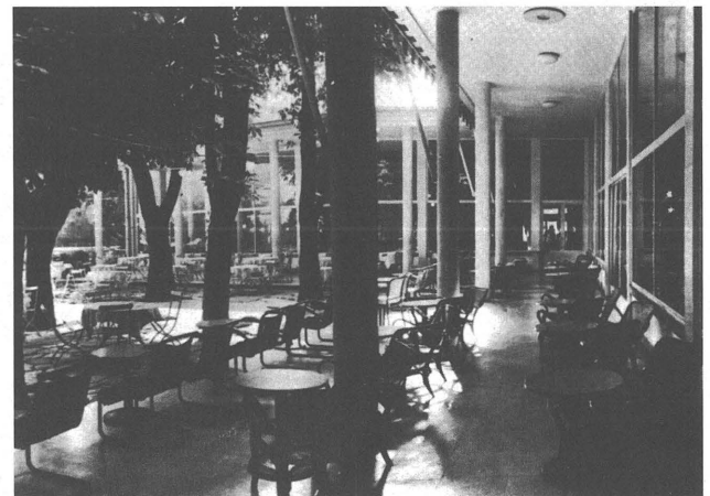
3.2. Café Greif in central Innsbruck, architect: Lois Welzenbacher, 1949/50. Photo: Albertina.
