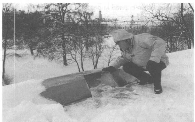
New copper flashing along the roof perimeter, at a downpipe.
