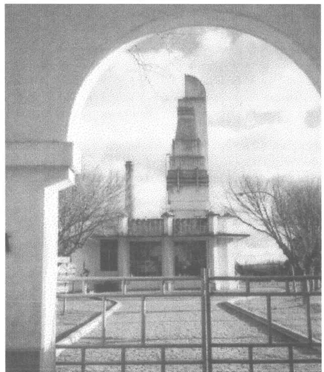
The Coronel Pringles slaughterhouse is today a designated landmark and used as a training centre. All illustrations courtesy of the authors.
