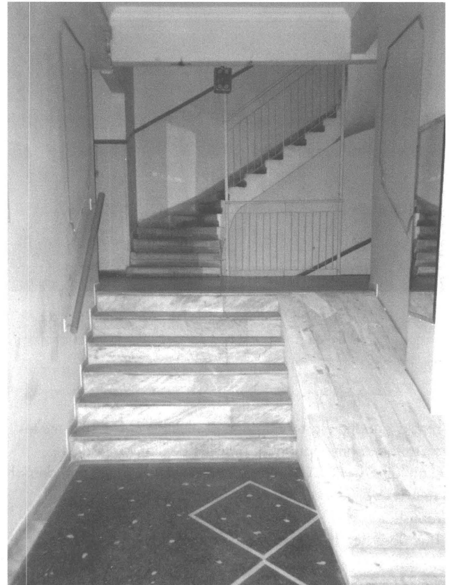
Typical apartment block entrance with the characteristic finishing materials like wood siding and marble flooring.
