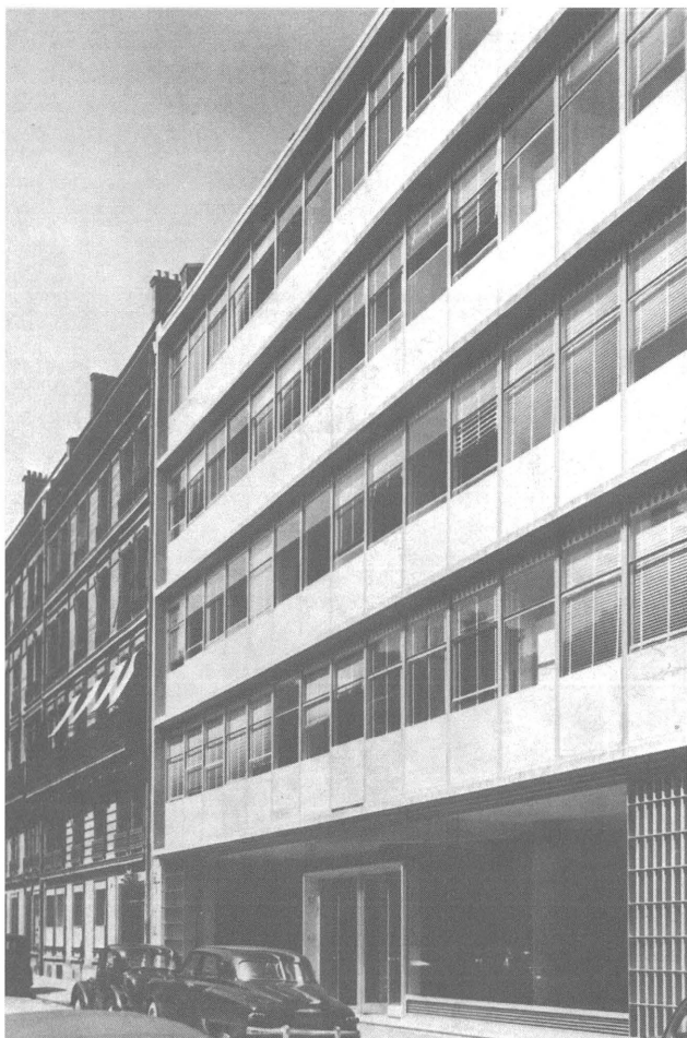
Left: The Fédération du Bâtiment in Paris (Prouvé, 1949), that involved floor-to-ceiling aluminium elements with vertical sash windows and a sophisticated ventilation system, has been key in the development of light aluminium facades. Photo taken from Jean Prouvé, Centre Pompidou , Paris 1990.
