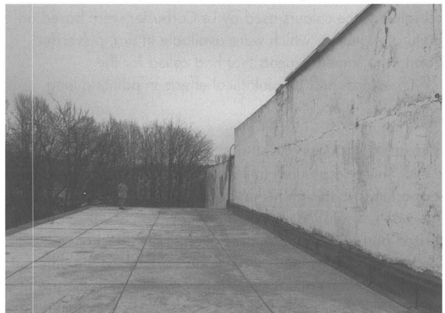
The roof in 2000, successfully repaired thanks to a Getty grant.
