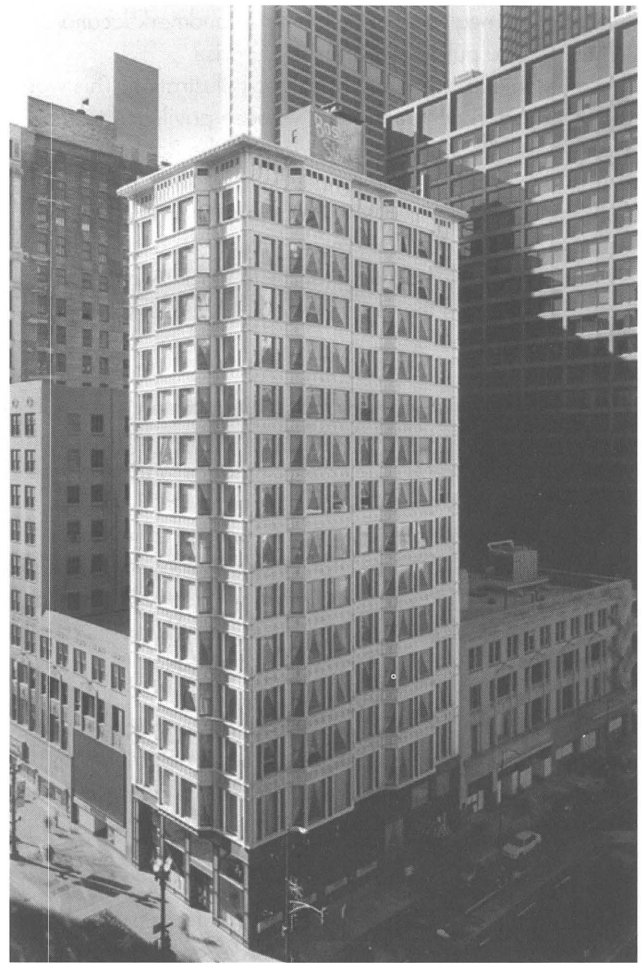
Chicago's Reliance Building, today the Burnham Hotel, has been carefully restored by DOCOMOMO-US vice president Gunny Harboe. Photo: Jon Miller of Hedrich Blessing.
