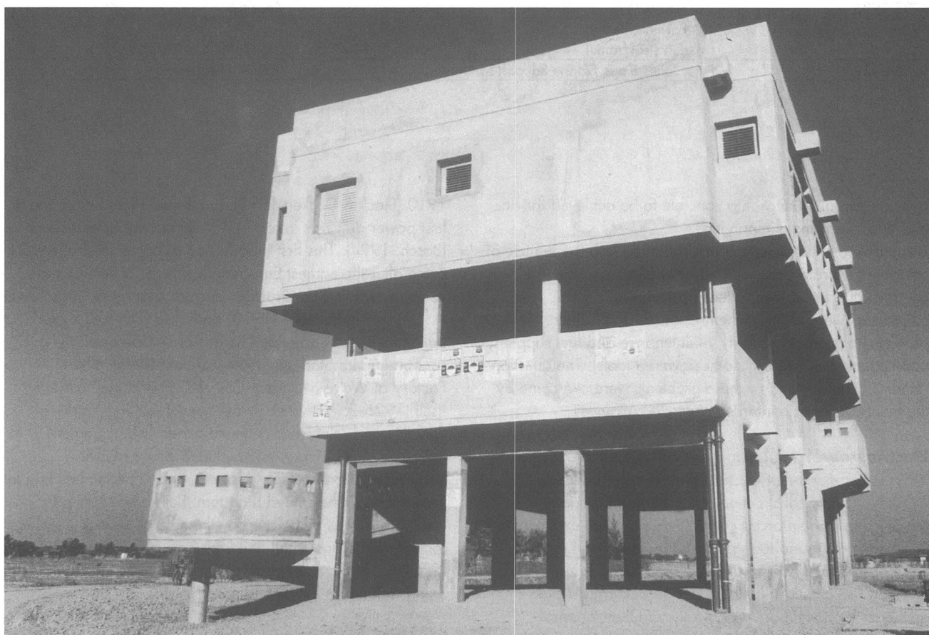
Cyclone-resistant concrete structures in Bangladesh. Photo: James Lewis.
