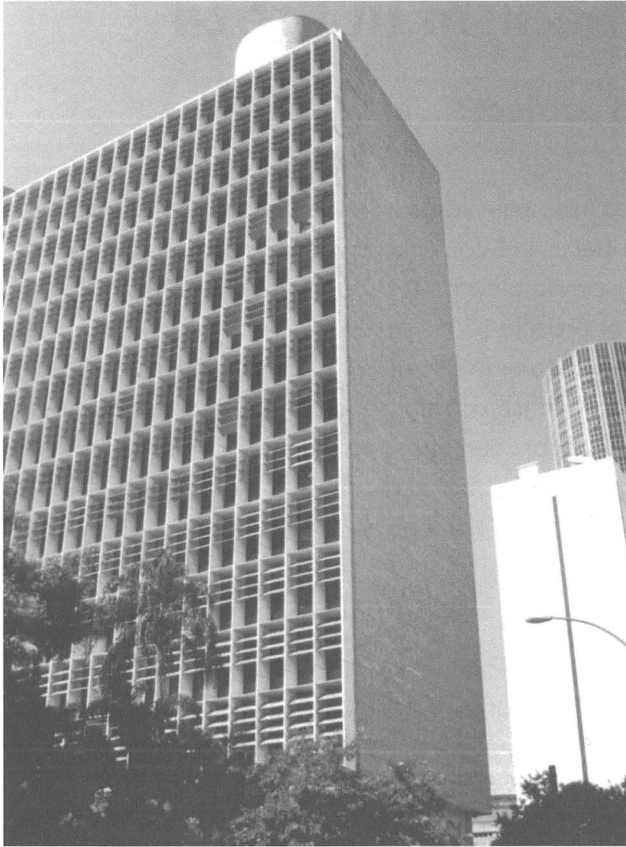
The creators of the Ministry of Education building, perhaps the most important single Modern Movement project in Brazil, argued that it should stand alone in the block, a guideline that was to be disrespected by Oscar Niemeyer himself when hired to design the commercial tower with the blank wall on the background of this photograph. Photo: V. del Rio.
