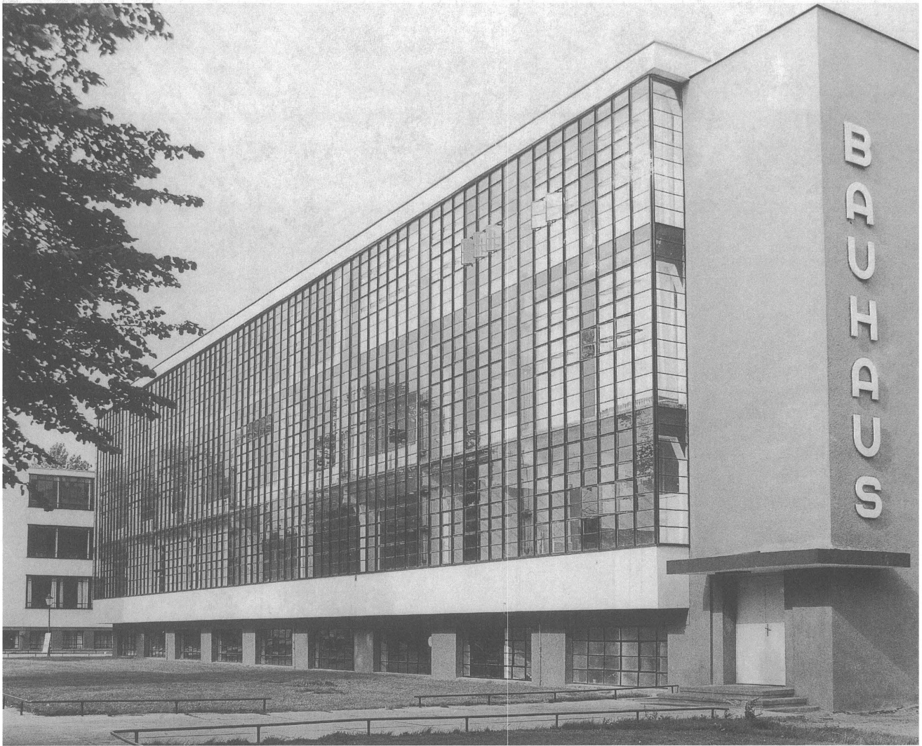
The Bauhaus Dessau curtain wall after the 1976 refurbishment.
