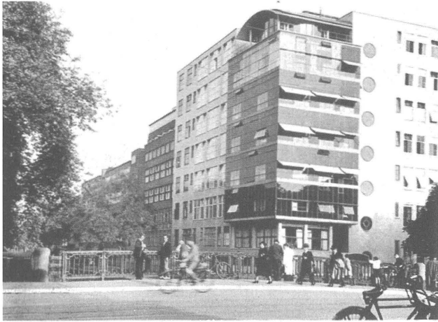
Amsterdam, 'De Joodsche Invalide', a large hospital visually integrated into the small scale of the canal district, J.F. Staal, 1935. Source: Wattjes, J.G., F.A. Warners, 1943, Amsterdams bouwkunst en stadsschoon 1306-1942 , Amsterdam 1943, 317.
