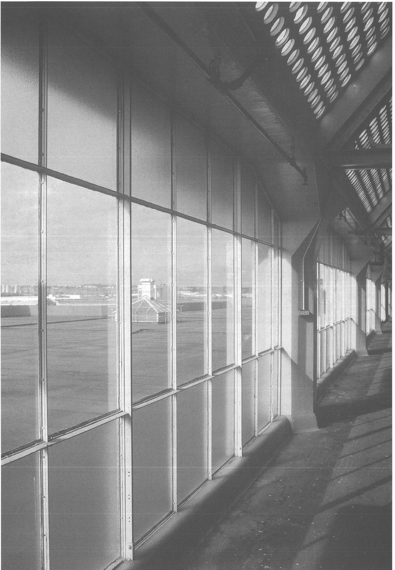
Inside view of Boots' curtain wall. Photo: Wessel de Jonge.
