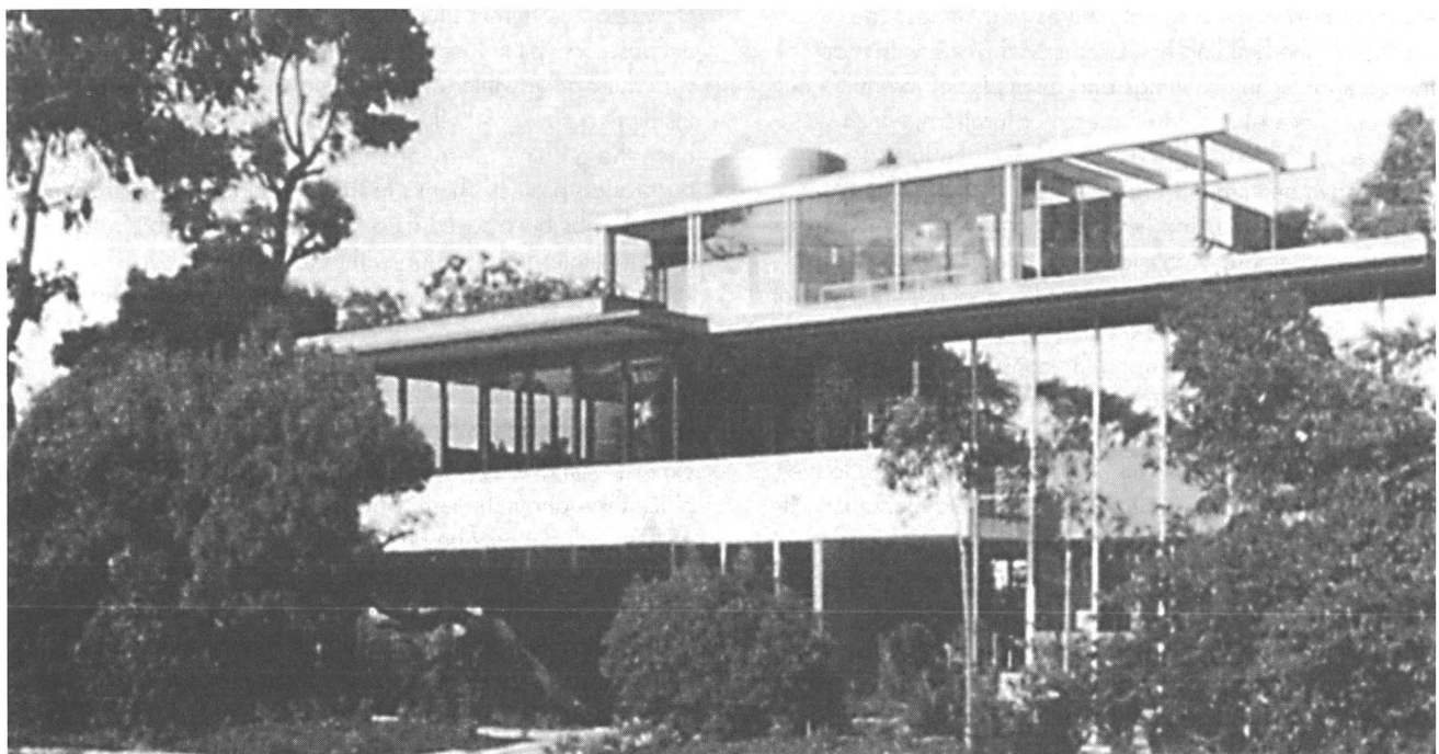
The rebuilt V.D.L. House, 1966.
