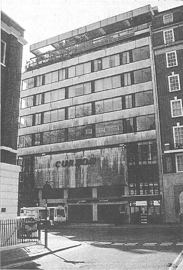
The Curzon Cinema, Central London, where the proposal to replace the aluminium framed secondary glazing with a tilt and turn pvc-u system, would have severely damaged the appearance of this listed building and meant the loss of a rare survival of a pioneering glazing system from the early 1960s.
