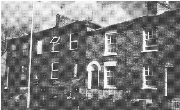
A typical conservation area whose appearance and character is marred by the replacement windows on the left. All photographs by courtesy of English Heritage.
