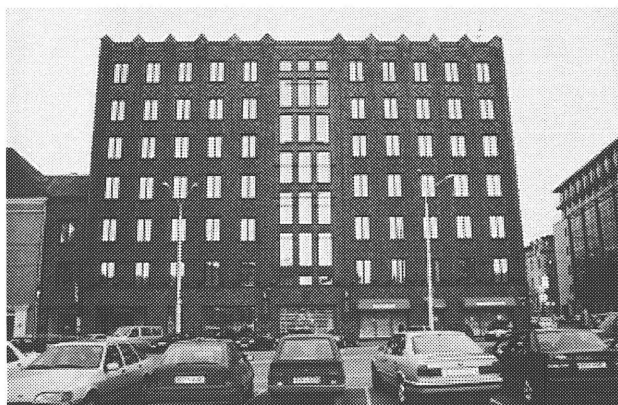
The front of the Tallinn City Government building, an outstanding example of Art Deco, changed into an expressionless face when pvc-u units were installed in 1994.
