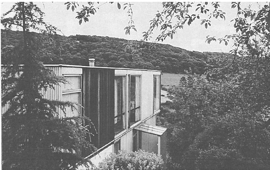
Aluminium-clad private residence at Almondbury, England by designer/builder Peter Stead (c. 1959). Photo: James Ashby.
