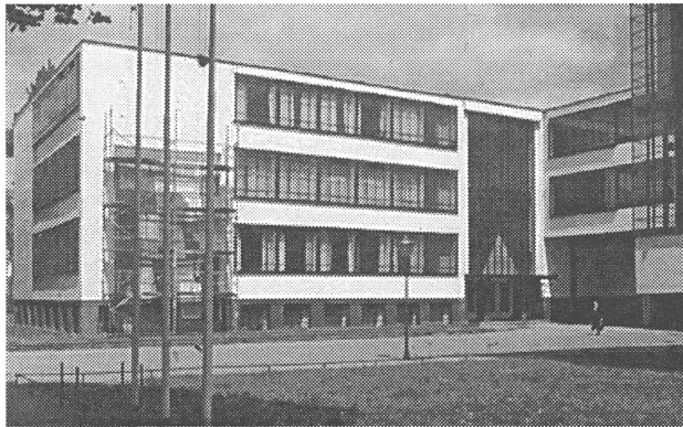
The Bauhaus Dessau school building (Gropius, 1925-26) in the present state, with the Municipal Technical School (left) and the workshop wing (right). The interior of the auditorium has been reconstructed. The replaced curtain wall has been a key issue when evaluating the building for the WHL in terms of meeting the test of authenticity.
