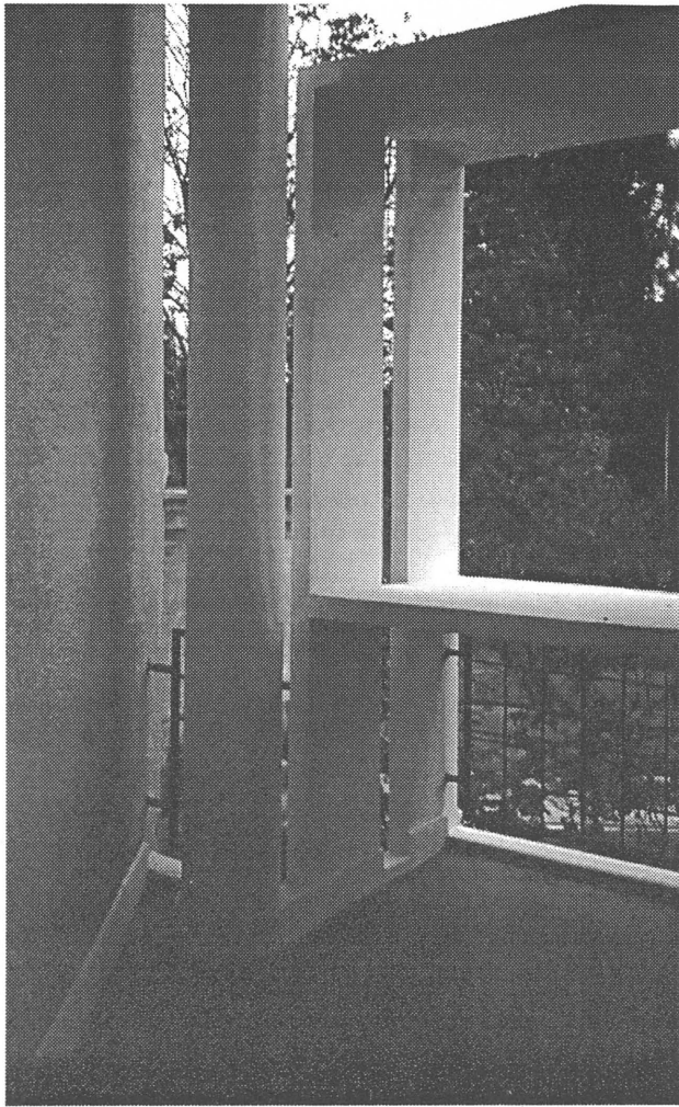
Detail of the sun screen showing the layered facade.
