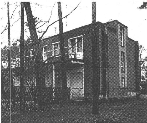
The Masters' Houses at Ebertallee 65-67 (Walter Gropius, 1925-26). Photo: M. Kuipers.
