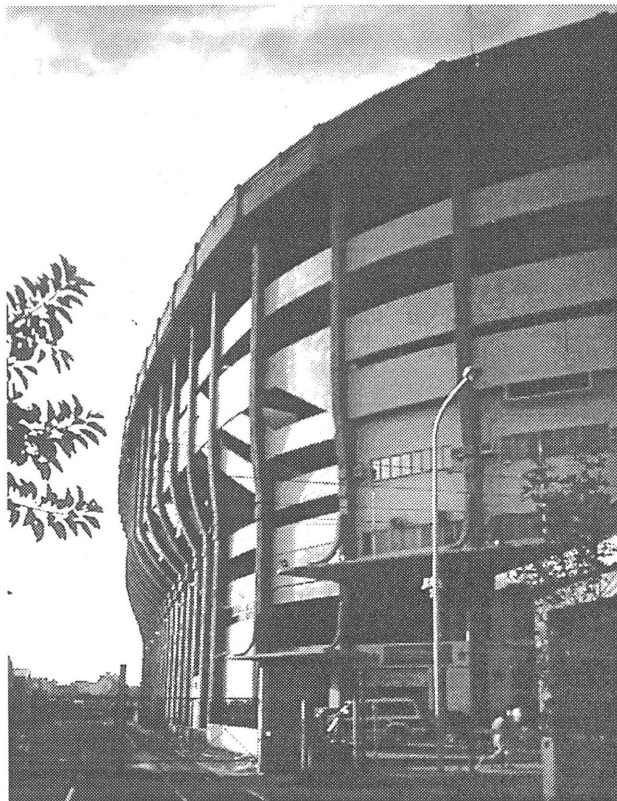
The third ring of La Boca stadium projects over the boundaries of the narrow site. Photo: Wessel de Jonge.
