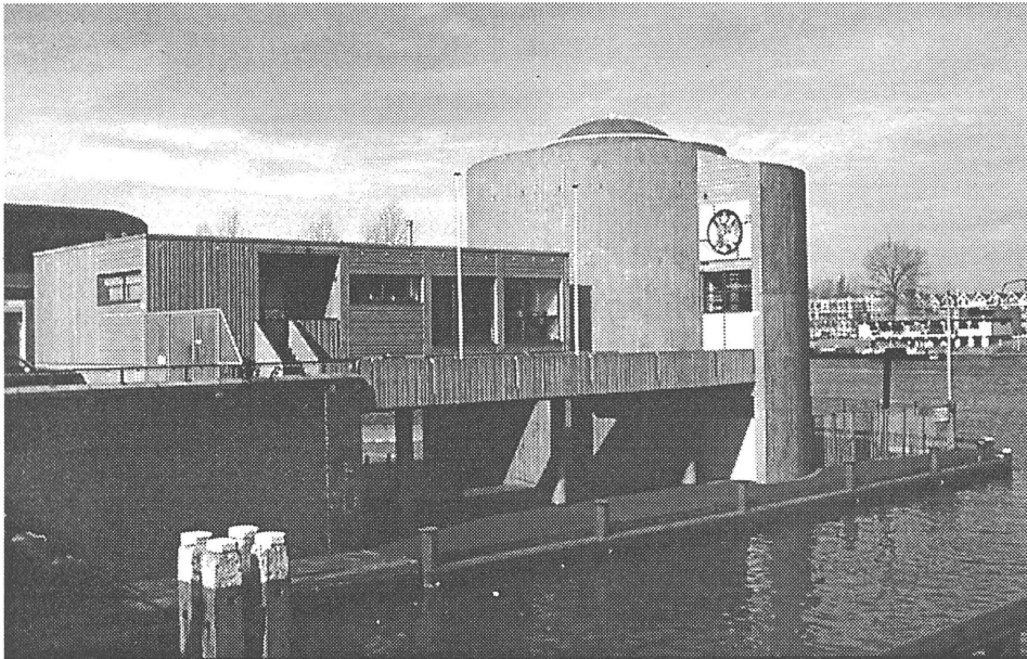
The pumping station seen from the nearby dike. The attendant's house creates a bridge to the engine hall. Photo: Wessel de Jonge.
