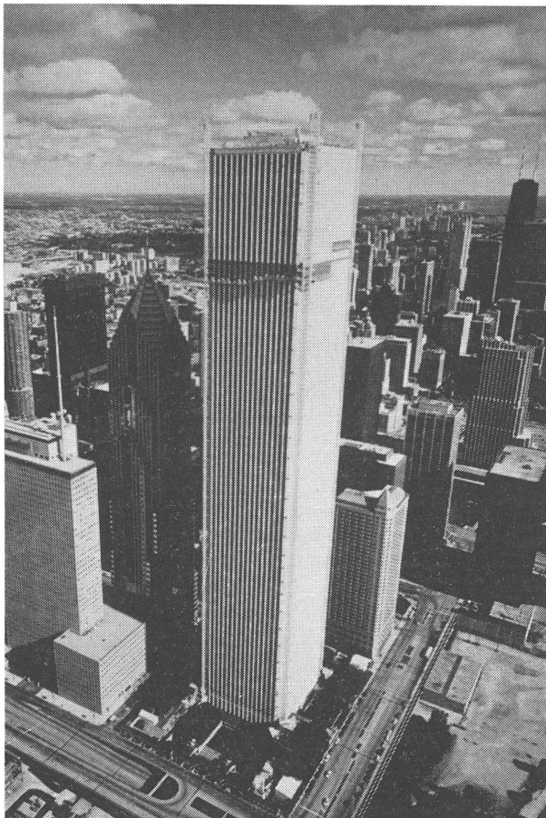
A view of the Amoco Building during recladding.
