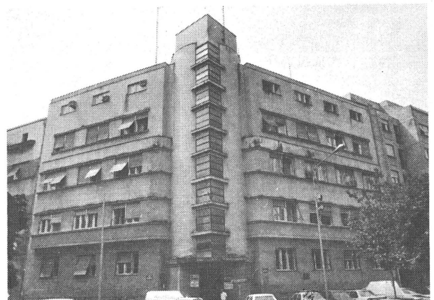
Building of the Yugoslav Daily in Novi Sad, 1932-36. Photo: Provincial Institute for the Protection of Cultural Monuments.
