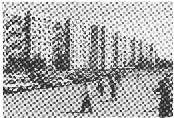
Top: panelsystem housing in the Purvciems district in Riga, Latvia.
