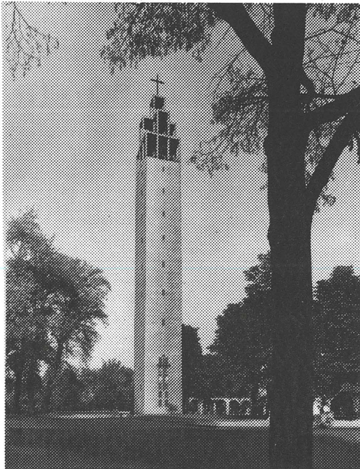
General view of the belltower of the Varosmájor church in Budapest, of which the particular top is being restored.
