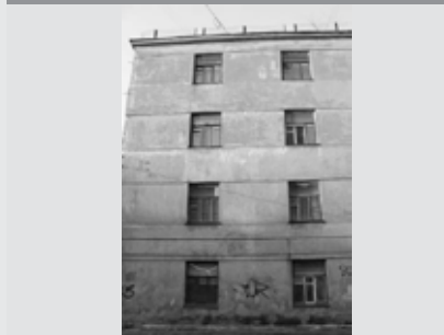
Figure 8. Dwelling, cleaned façade
