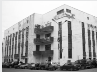
Figure 3. Administration building. Before 1932
