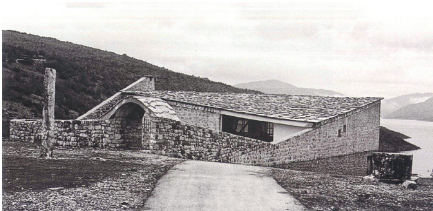
Historic view of the Regional Museum at Bileća lake ethno-park, around 1975. © Tatjana Neidhardt, Juraj Neidhardt's private archive.
