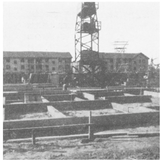
07 First silicate block building in construction in Shanghai. © Architectural Journal, 1960 (03), p. 3.
