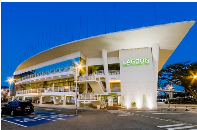
07 The original design turned into a monolithic block housing a shopping mall, hiding the view to the lagoon and extinguishing the monumentality of the pillars. © Riotur, Verônica Peixoto, Year.
