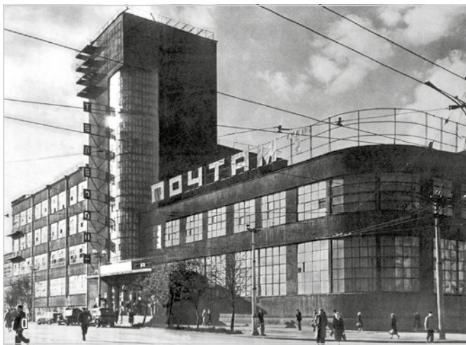
09 (a) The Post Office Building. © Unknown, 1930s. (b) © Chahovets, 2020.
