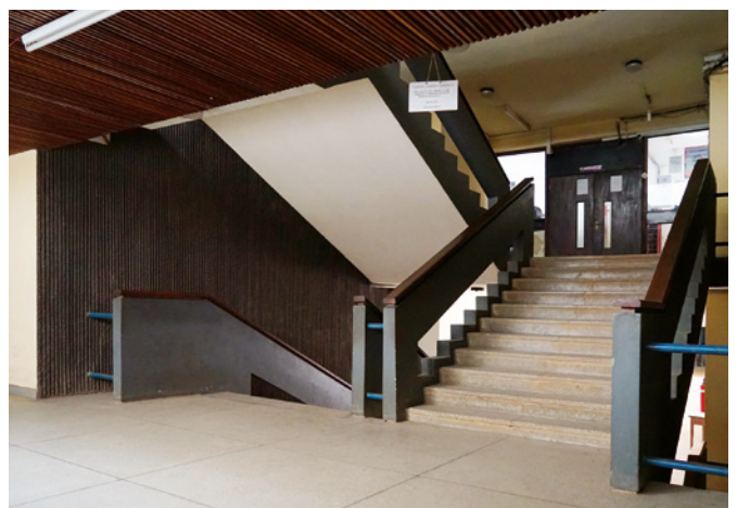
18 Obafemi Awolowo University, Library, circulation area with terrazzo flooring, raked spray render wall surfaces, wooden ceiling cladding and handrails, painted concrete, blue metal railings, 2022. © Brenne Architekten, 2022.
