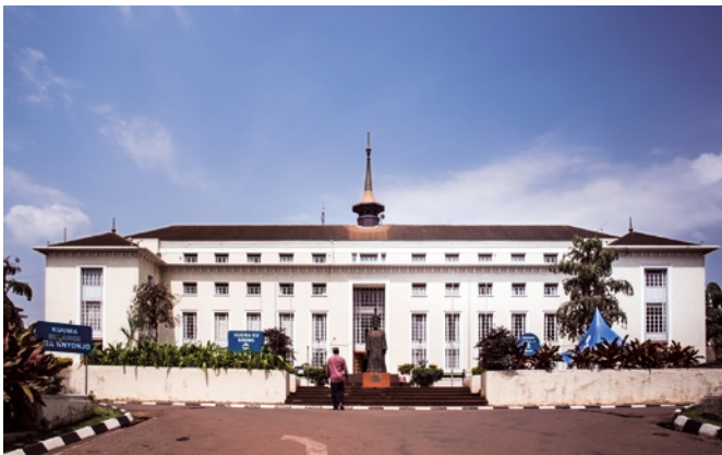
03 Front elevation of the parliament and offices of the Buganda Kingdom, the Bulange. © Timothy Latim 2018.
