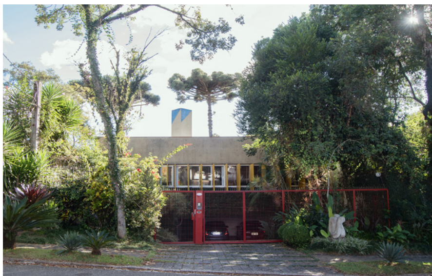
01 Manoel Coelho's house, front facade. © Author, 2022.
