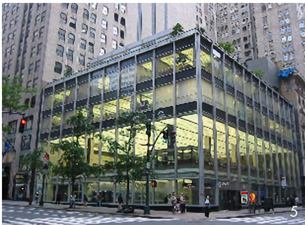
Figure 5. Gordon Bunshaft (SOM), branch bank (formerly Manufacturers Trust and most recently Chase), New York, 1954. In the second floor banking hall a screen designed by Harry Bertoia is partially visible from the street. Photo by Theodore Prudon.
