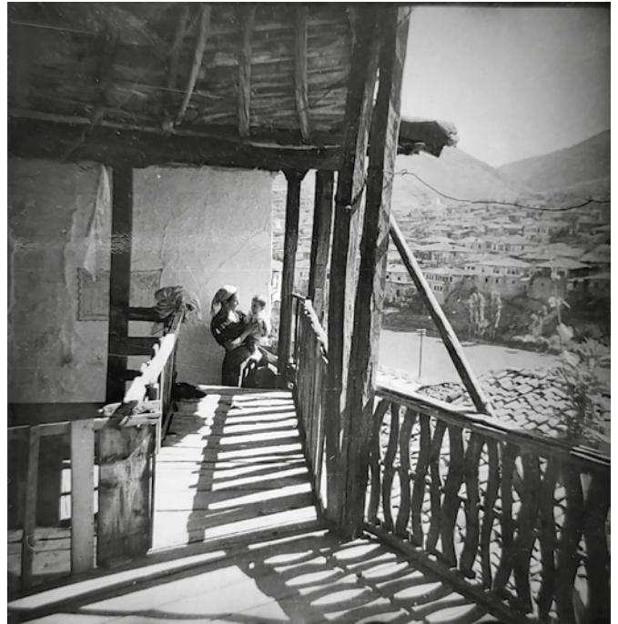
07 The spatial journey between the stairs linked to the čardak by an open bridge, and from all these spaces a connection to the outdoor and public realm. Note the openness of the liminal space between the closed private rooms and the exterior, Veles, 1947-1949 © Photograph by the Grabrijan and team, 1947-1949, Grabrijan archives (Folder 4, drawer 5.2: Macedonian House), Museum of Architecture and Design, Ljubljana.
