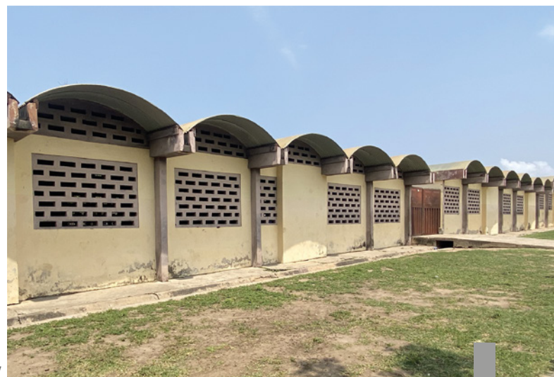
06 Façade of Republic Road School showing the use of repetition of roofs, breeze blocks, and columns. © Author, 2022.
