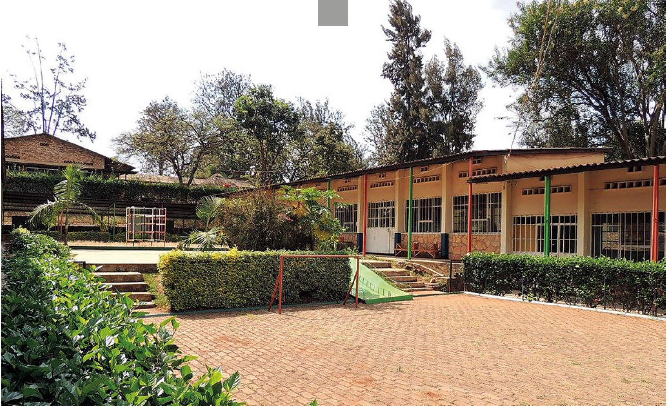
02 École Belge showing a front view of one of the classroom blocks. The walls and structural columns of the blocks follow a logical pattern of repetition, creating a rhythm on the façade. © École Belge de Kigali, 2015
