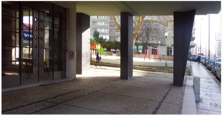
05 The blocks are standing on pilotis with a marble finish. © Ana Vaz Milheiro, 2023.
