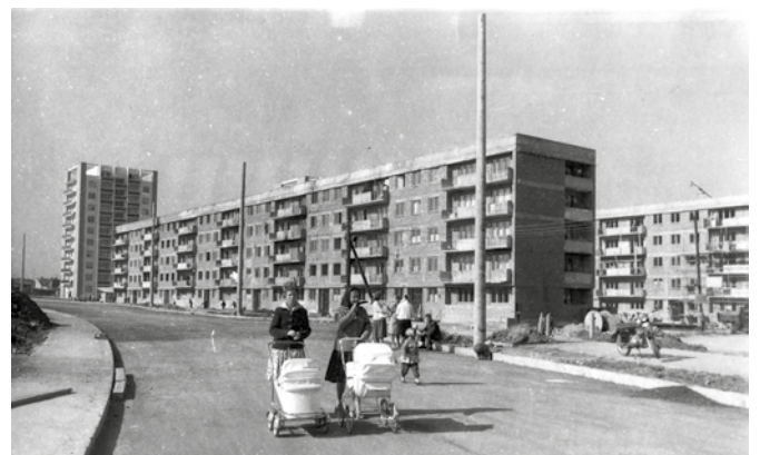
10 Construction site, microraión 1, Gheorgheni housing estate, Cluj. © N. Kulin, April 1965, DSAPC Cluj.
