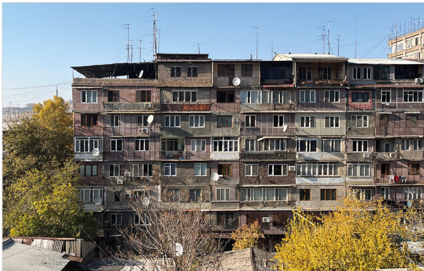
04 A mass residential building in Yerevan with an added top floor and individually glazed balconies. © M. Karaselnikova, 2022.
