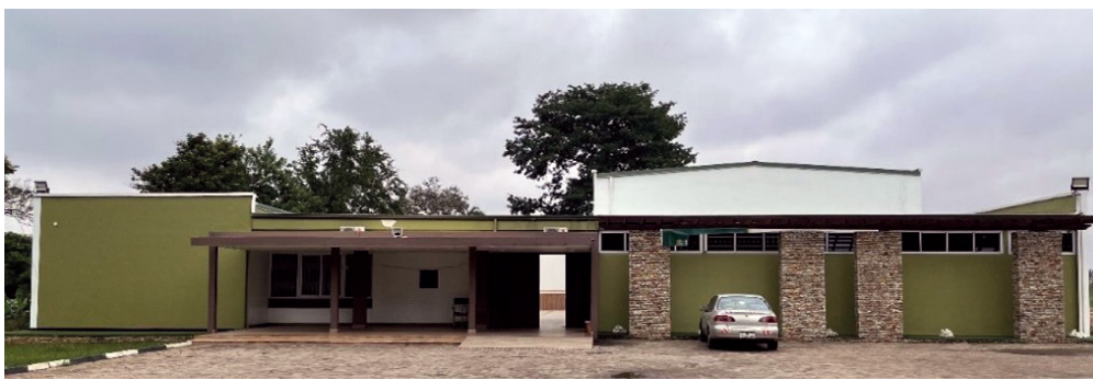
06 KCC after renovation, front view towards entrance and view of open court. © Author, 2023.
