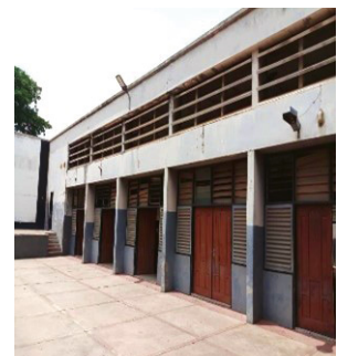
02 View of closed 'dry' court at KNUST Community Center. © KNUST Development Office, 2023.
