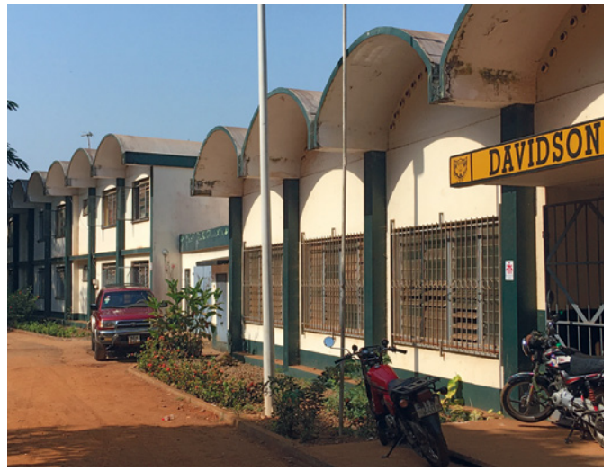
09 Halls of Residence. © Paul Robinson, 2023.
