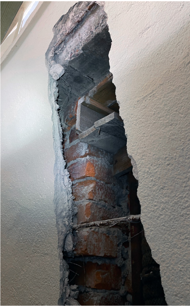
08 The rotunda wall intervention provided access to existing pipes for renovation purposes, while also revealing the wall construction and multiple layers of the wall's unique rendered texturing for research purposes. © Marcelo Rovira Torres, 2022.
