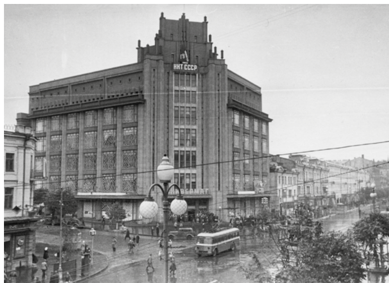
07 Kyiv, Khreshchatyk Street 38. Building of the Central Department Store (TsUM). © Unknown, photo from the 1970s. Central State Film and Photographic Archives of Ukraine.
