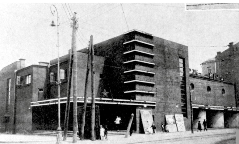
08 Kyiv, Kostyantynivska Street 26, "October" cinema by architects N. Trotsky and V. Rykov, 1928-30. © Unknown, original photo, Building of Socialist Kyiv - K., 1930.
