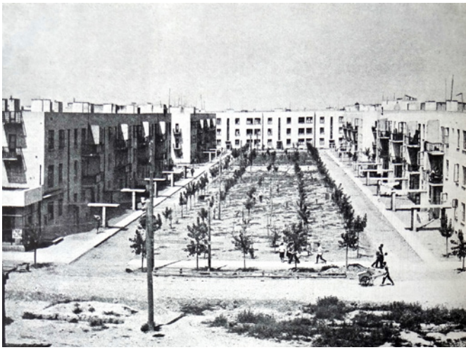
06 The 6th settlement in Zaporizhzhia. VIII quarter. © Unknown, from the early 1930s, Arkhytektura SSSR (1933), 3-4, p. 36.
