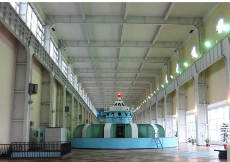
05 Interior of the hydroelectric station. © S. Smolenska, 2017.
