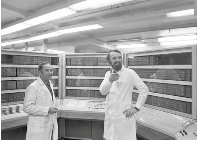
04 a KyivZDNIIEP, computers, architectural engineers. © Viktor Maruschenko, courtesy of Alex Bykov, 1983.
